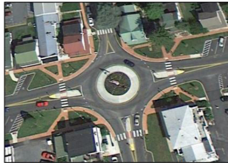
(Source: PennDOT Local Technical Assistance Program)
