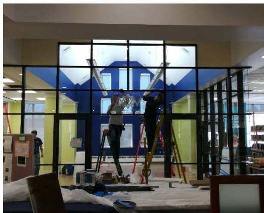
Workers install glass in the NOW Lab
