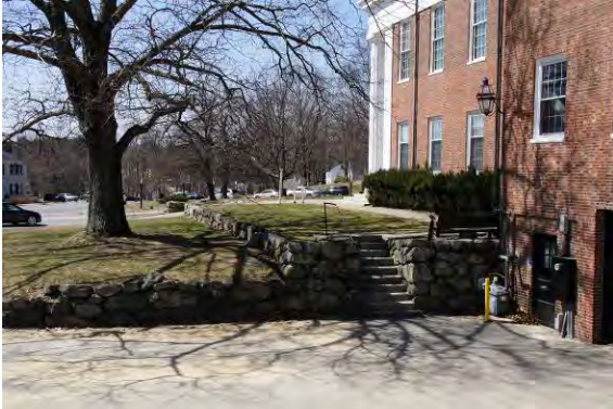
Figure 74. Stone retaining wall on south side of Town Hall with stairs leading up to the Town Clerk door.
