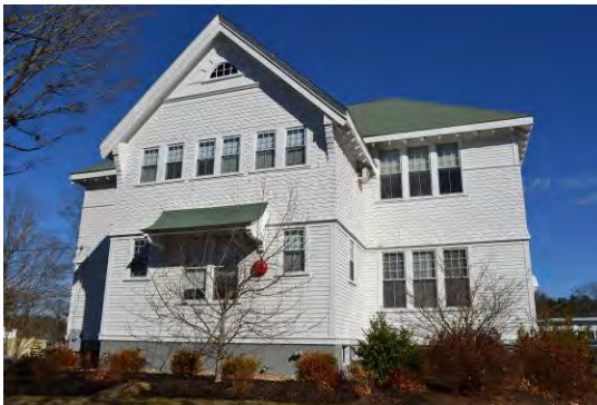
Flynn building west elevation from Old Sudbury Road
