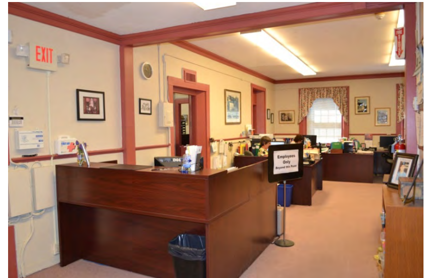
Raised concrete floor at Town Clerk office should remain
