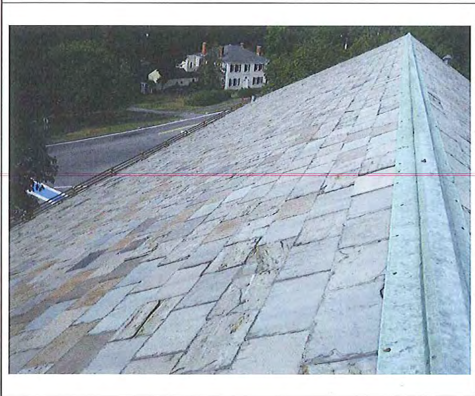
Photo No. 02 Location: Sudbury Town Hall Description: Overview of slate roof.
