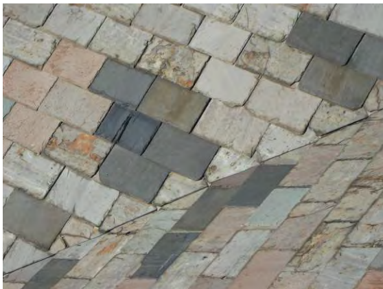
Figure 23. View of slate valleys and slate condition.
