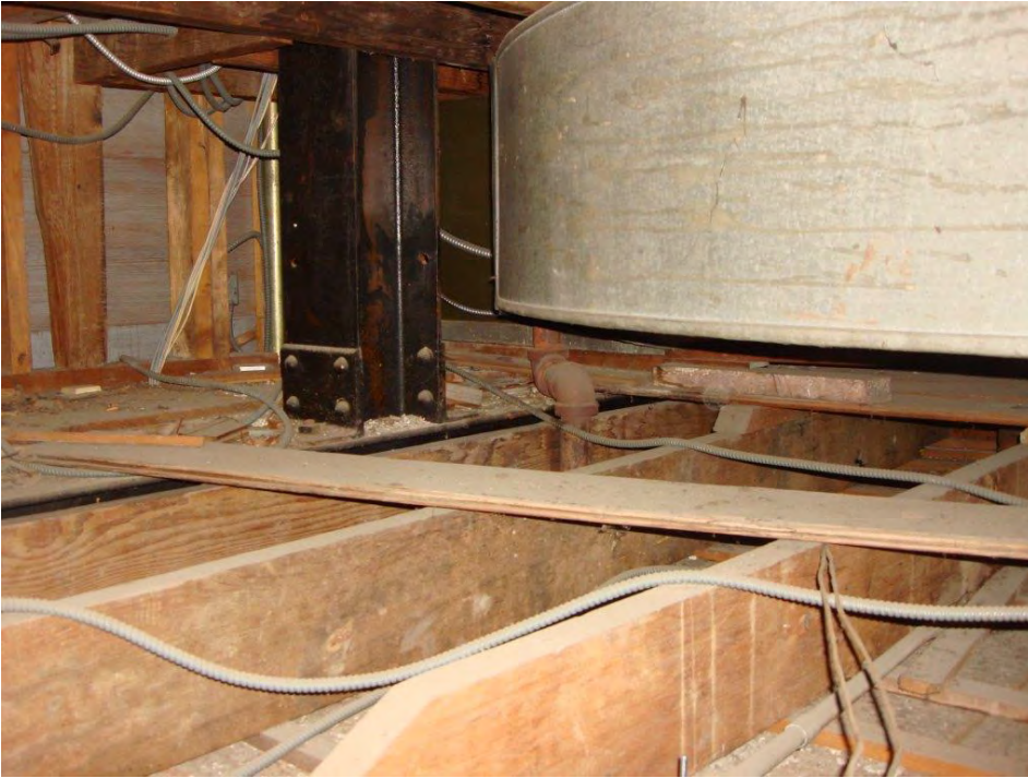
Steel proscenium column supported by beam
