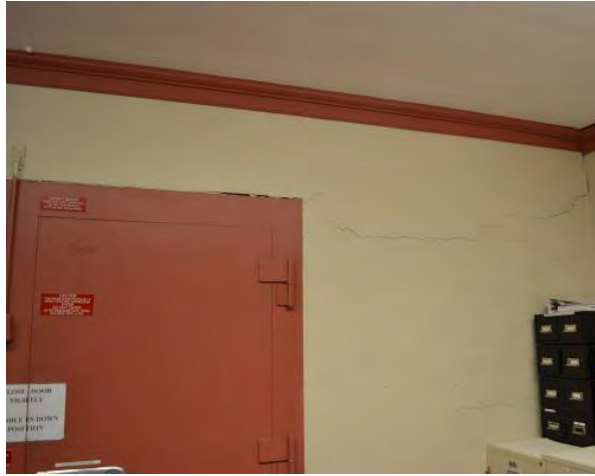
First floor vault in Town Clerk's office (Town Hall)
