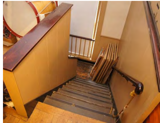
Figure 52. South balcony stairs
