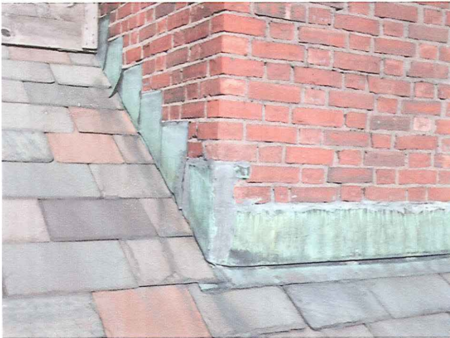
COPPER FLASHINGS @ LEFT SIDE CHIMNEY
