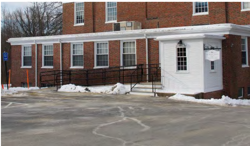
Figure 43. East entry stair and ramp to Town Clerk.
