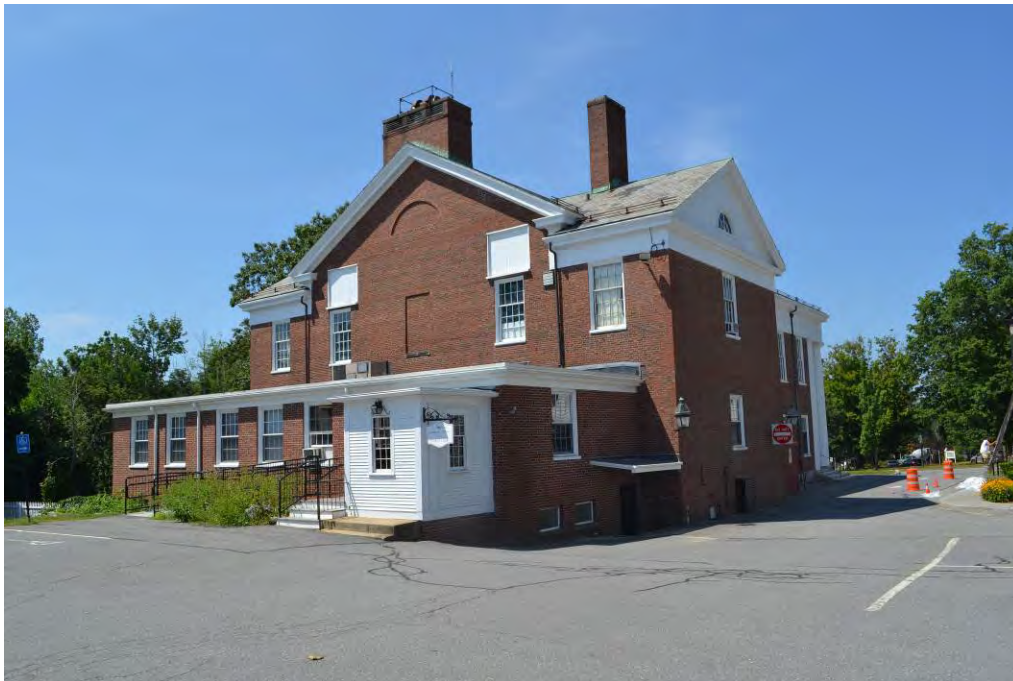
Figure 5. Sudbury Town Hall east façade.
