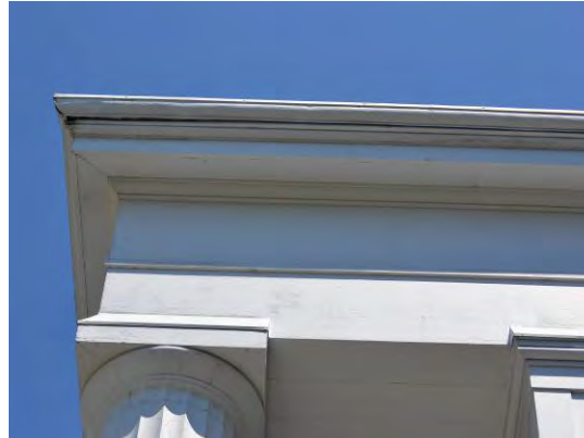
Figure 28. Wood trim around exterior walls.
