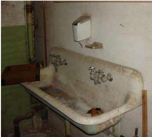
Figure 61. Old sink in basement.
