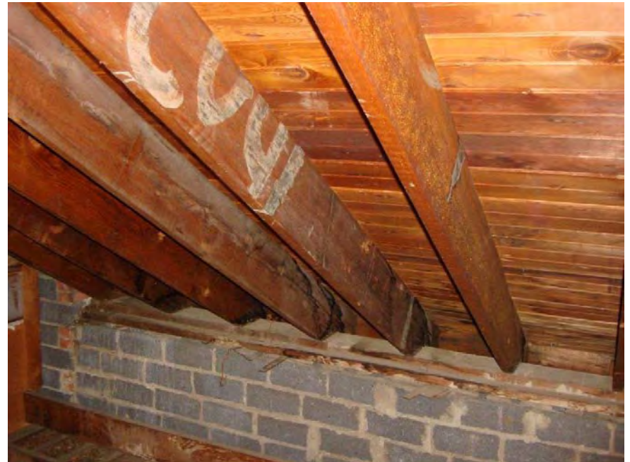
Existing roof rafters at cinderblock exterior wall
