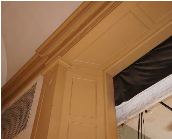
Figure 46. Proscenium trim and paneling.
