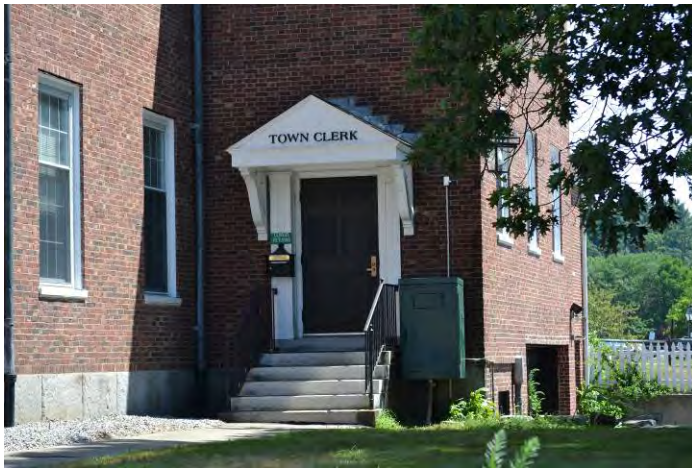
Figure 40. South wing entrance door to Town Clerk's office.
