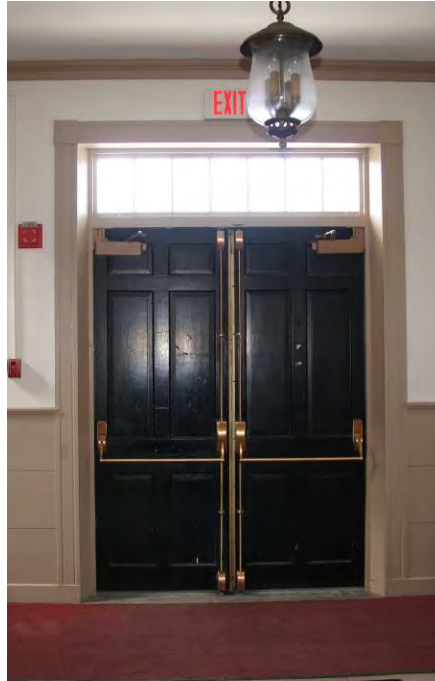
Figure 39. Interior of entrance doors.
