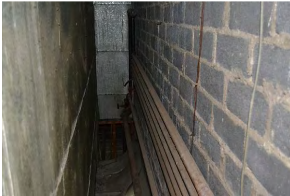
Figure 27. Cinder block at exterior wall behind stage.
