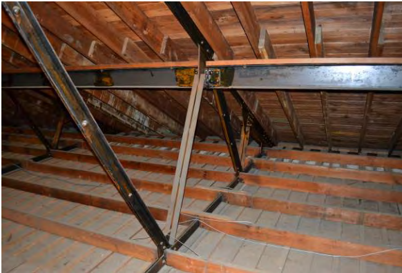
Figure 18. View of auditorium ceiling framing, steel truss and steel beam.
