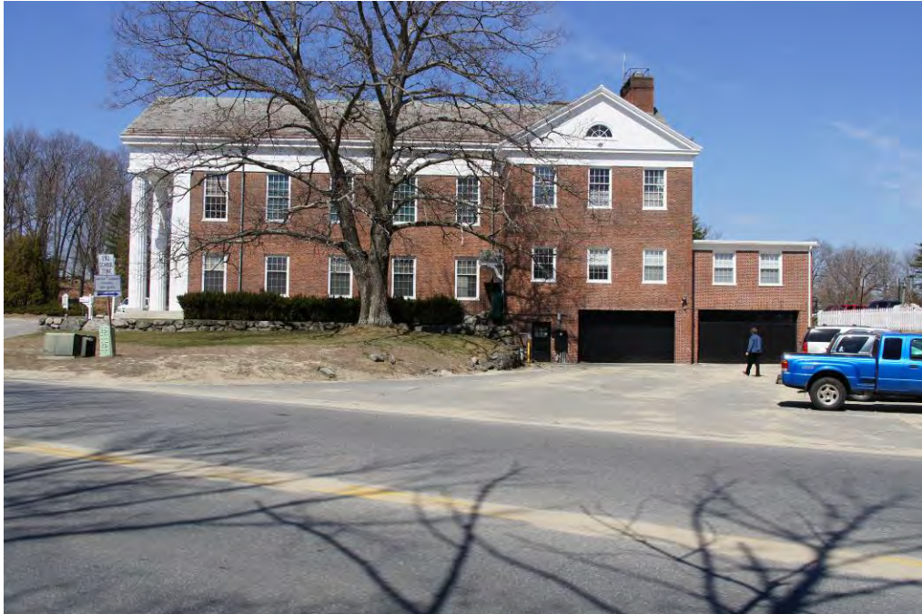
Figure 4. Sudbury Town Hall south façade.
