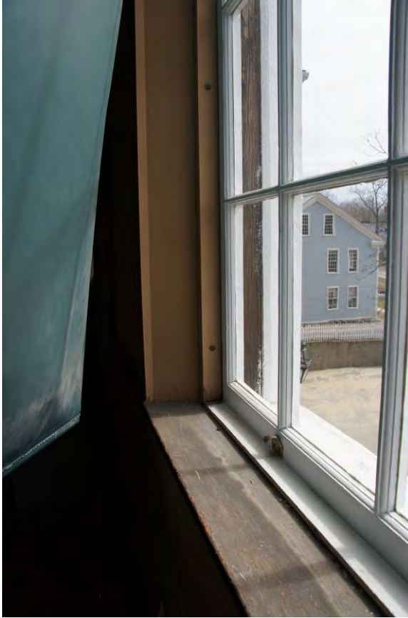
Figure 37. Restored original wood window on the south elevation.
