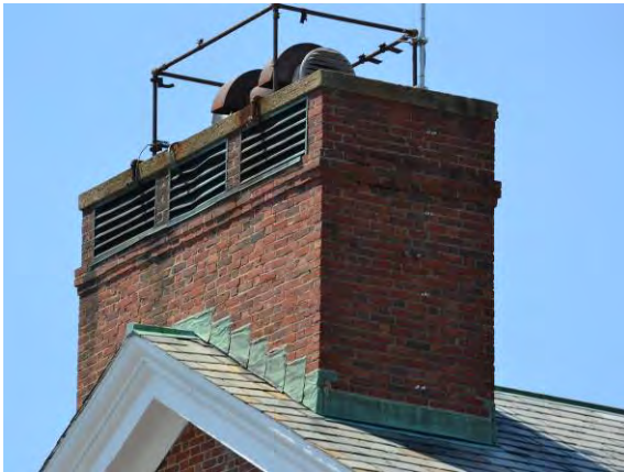
Figure 29. East chimney above roof.
