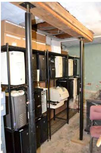
Added supports in basement
