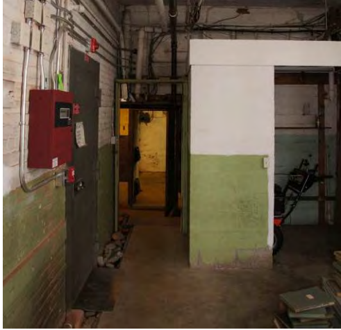
Basement vault in Town Hall
