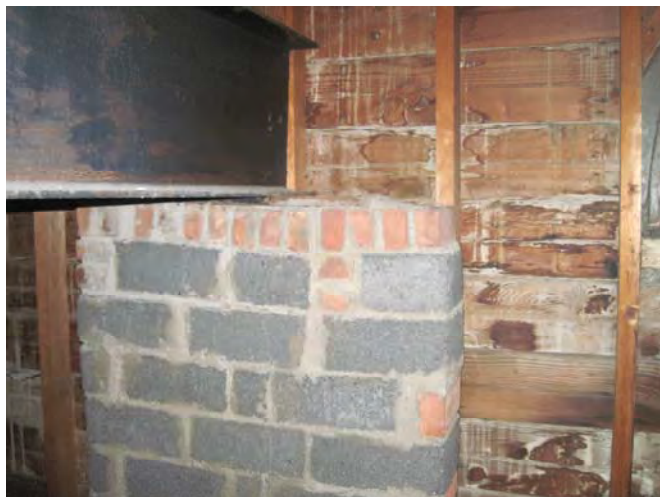
Figure 5-Masonry Pier Supporting Attic Beam (North Side Gable)
