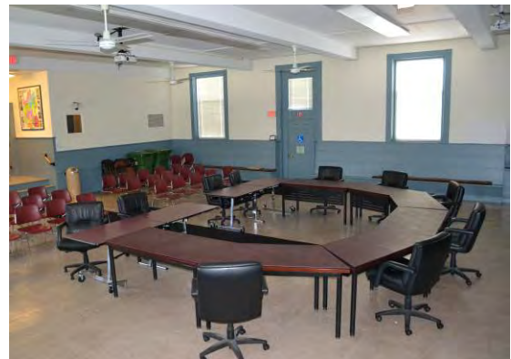
Figure 59. Vinyl tile on floor, plaster on walls, and acoustic ceiling tiles at meeting room.
