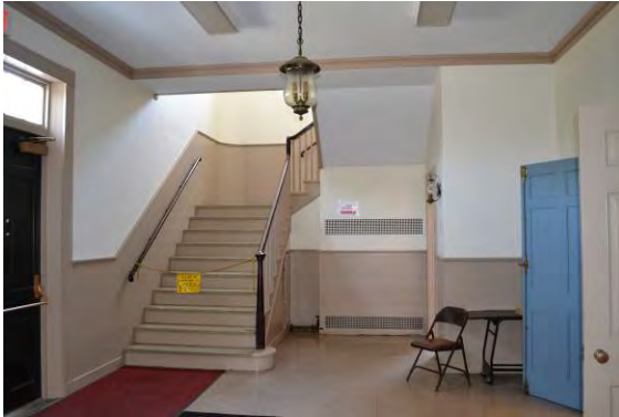
Figure 49. North stair in main vestibule
