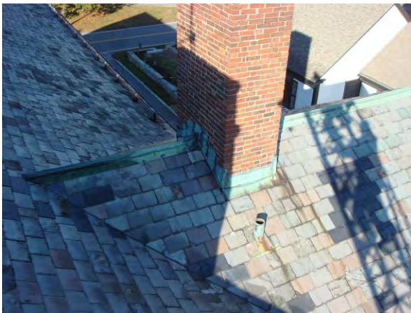
Figure 31. North chimney above roof.
