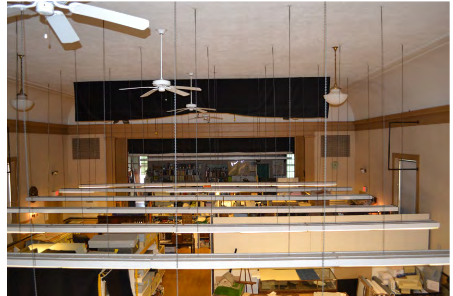
View of auditorium from mezzanine
