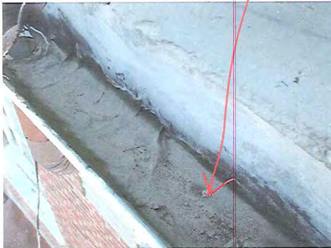
COPPER GUTER LINED W/ TAR
