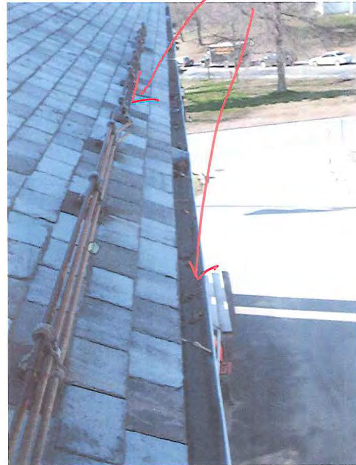
VIEW OF LEFT SIDE SNOW RAIL & GUTTER
