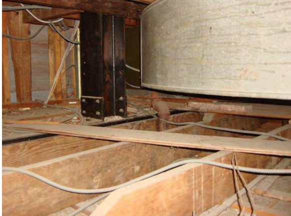
Figure 15. Steel proscenium column supported on beam under stage.
