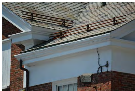
Figure 21. View of painted copper gutters and snow guards at northeast corner
