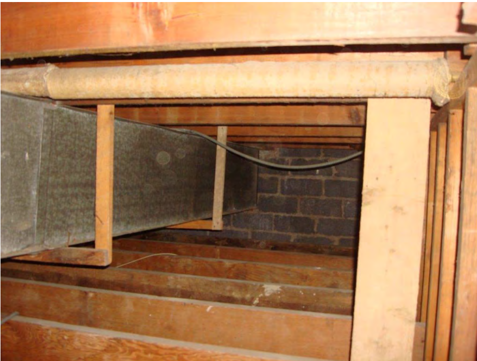
Stage floor and 1 st floor ceiling joists at cinderblock exterior wall
