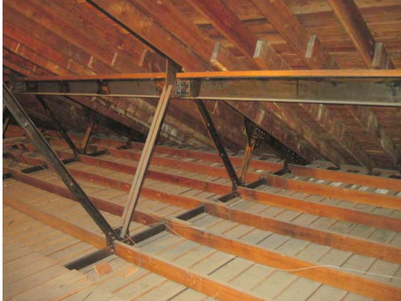
Figure 4-Auditorium Roof Truss and Rafter Framing
