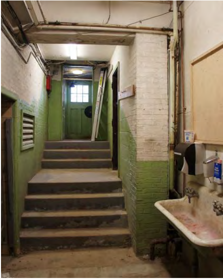
Figure 12. Stairs leading to the north exterior door in the 1955 addition.
