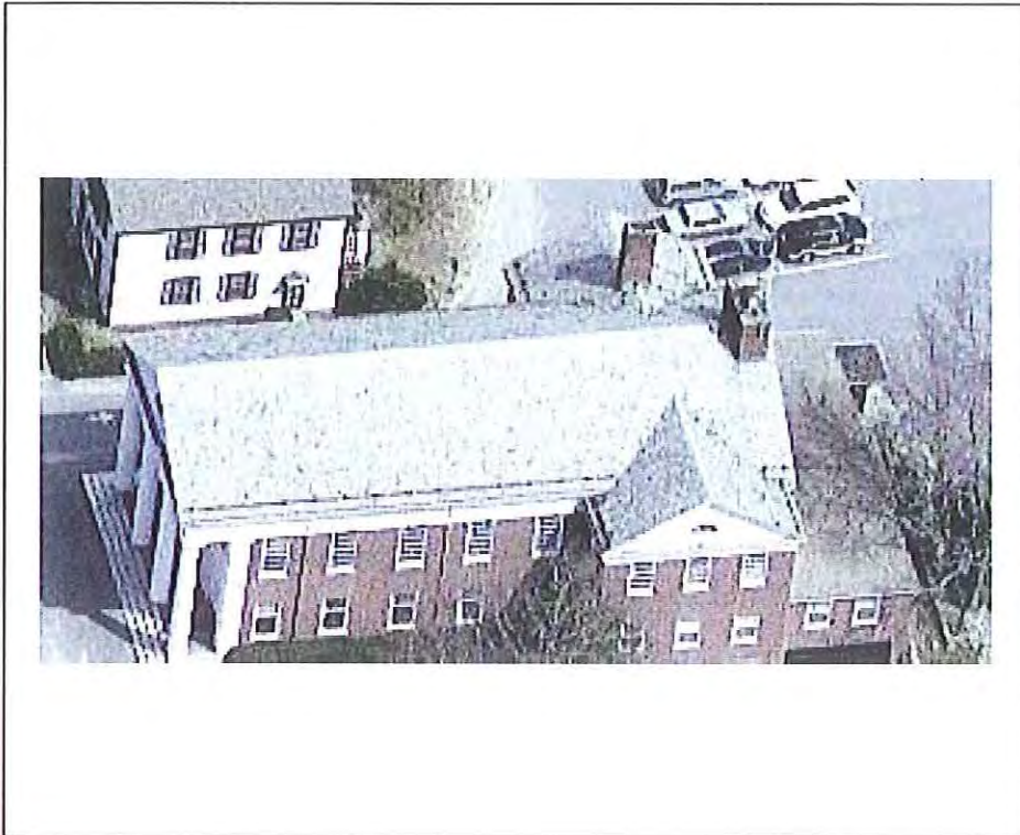
Photo No. 01 Location: Sudbury Town Hall Description: Aerial View of Roof.
