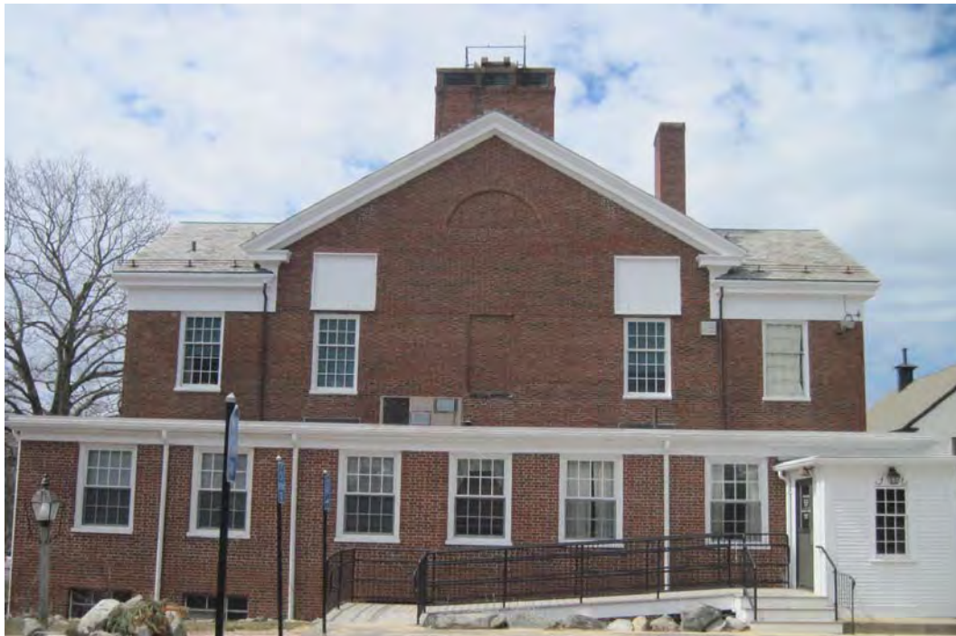
Figure 6-1955 Addition at Rear of Town Hall
