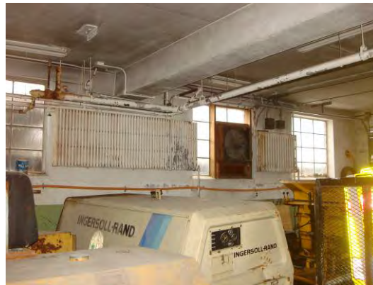
Figure 11. 1955 fire station bay. Note concrete beam supporting floor above.
