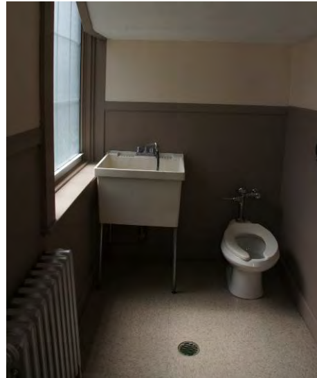
Figure 55. Men's restroom at front vestibule.
