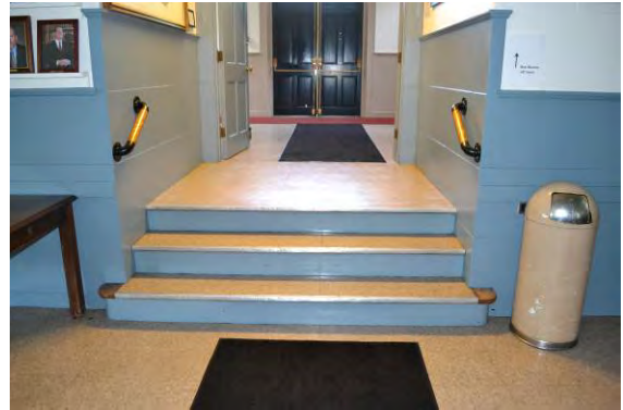
Figure 50. Three stairs down from vestibule to meeting room
