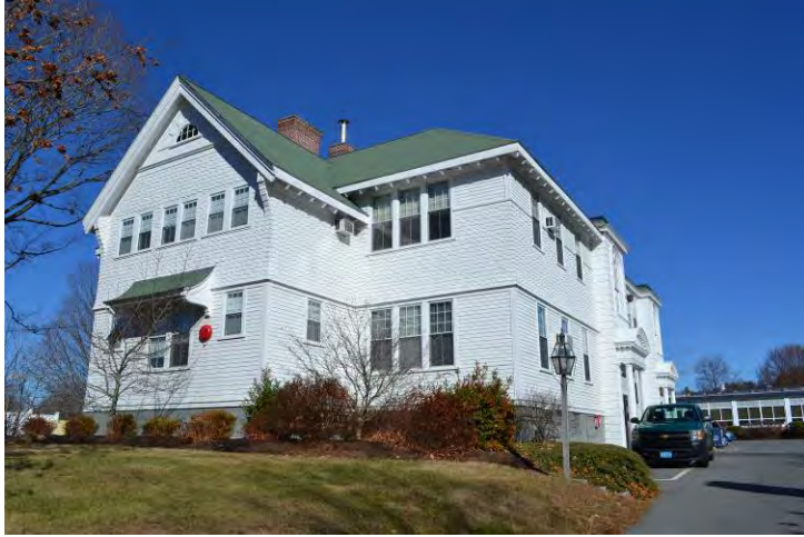
Exterior of Flynn Building
