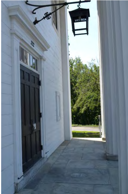
Figure 38. Front entrance doors under portico.
