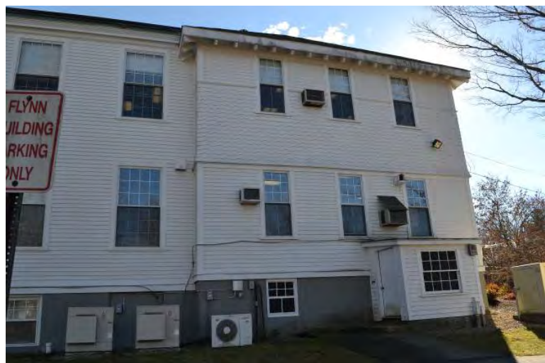
Window and wall air conditioning units and supplemental air conditioning units
