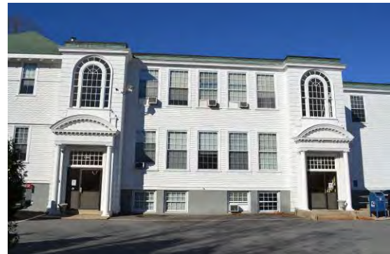
South elevation of two entrances
