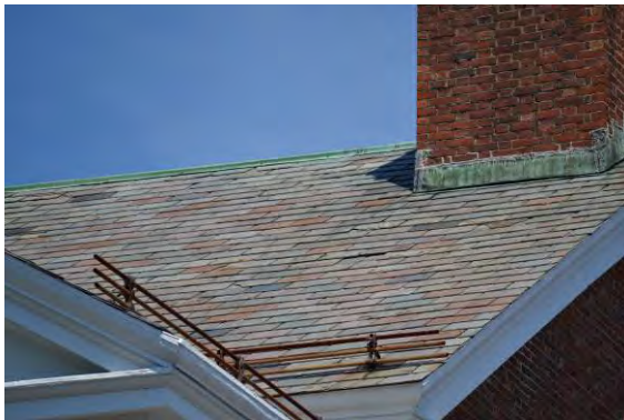
Figure 20. View of slate at southeast corner
