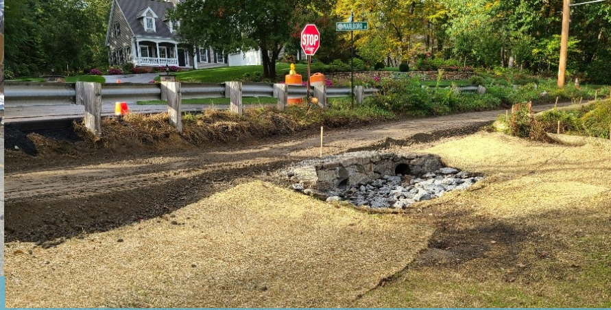
WORK IN PROGRESS: New drainage, asphalt berm and preparations for paving walkway.
