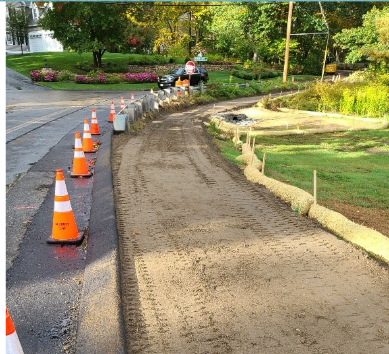
WORK IN PROGRESS: Grading preparation for walkway, soil stabilization and new stone headwall.
