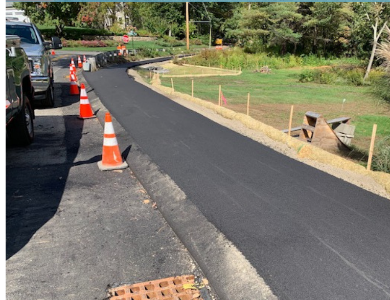
WORK IN PROGRESS: Morse Road walkway complete.
