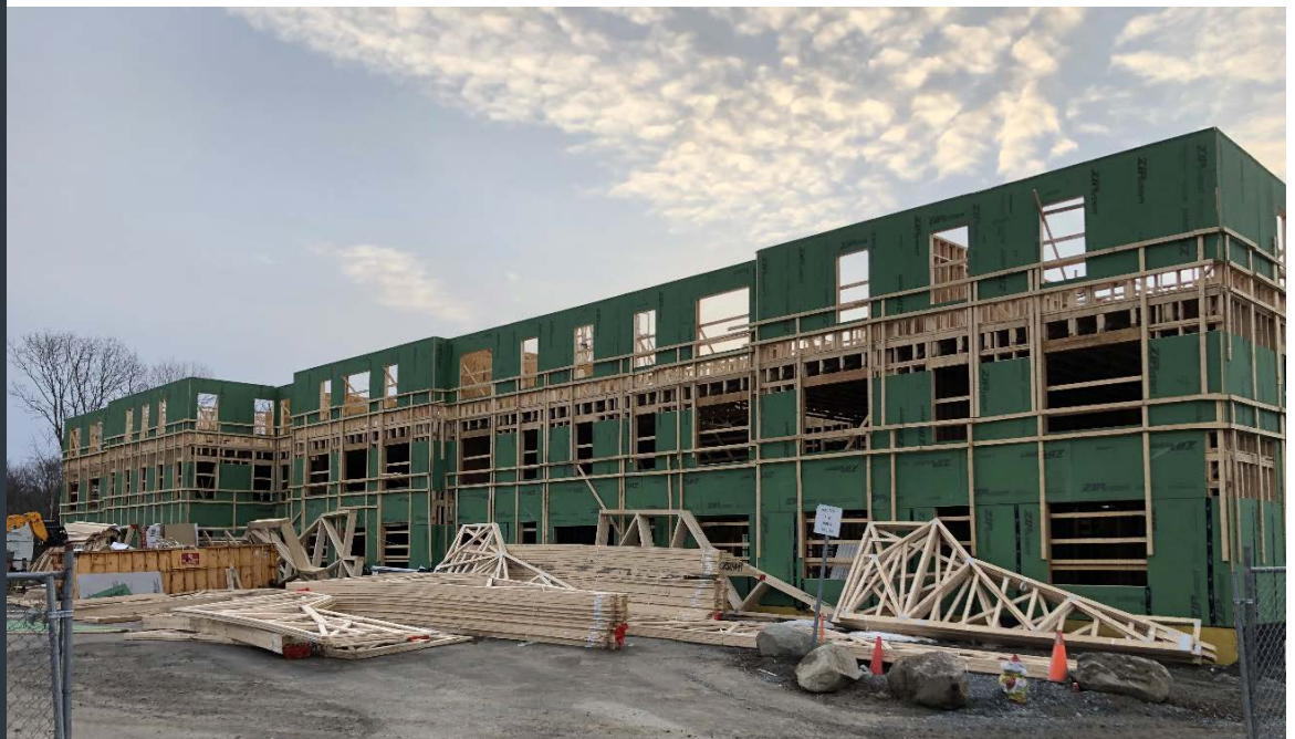
Construction at Coolidge Phase II
