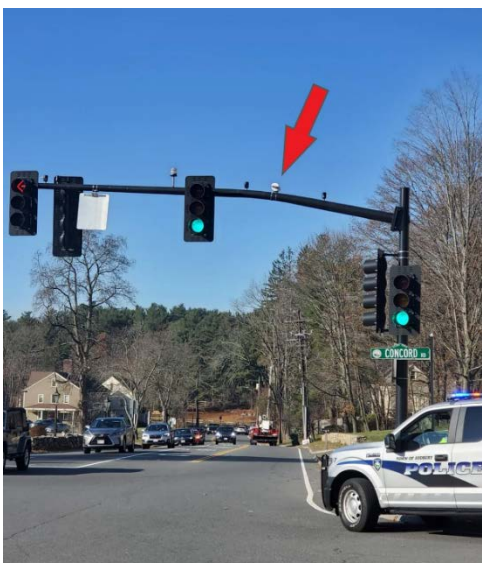
RWIS monitors provide the DPW with information on pavement conditions that helps make winter roadway treatment more efficient.
