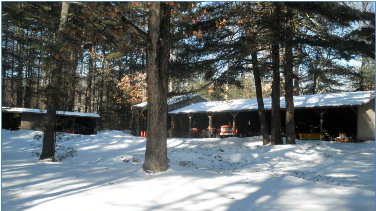
Photo #4 – Open-bay maintenance garage – typical of accessory improvements.
