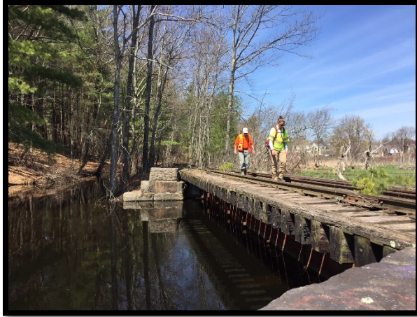
Eversource site work preparation.
