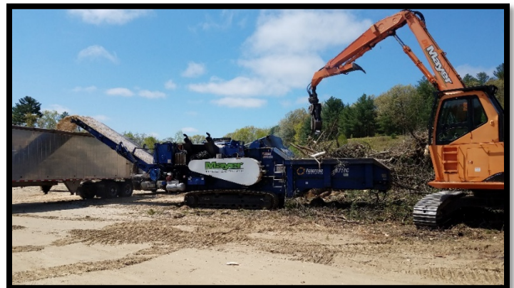
Town-wide removal of debris resulting from the winter storms that battered Sudbury this winter has wrapped up. Pictured above is the chipping of the debris that took place at the Melone property on Route 117.
