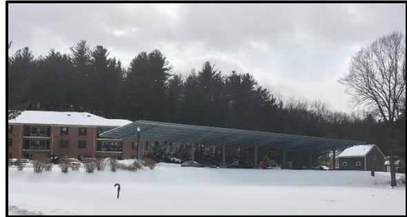
The new solar carport at 655 Boston Post Road (Longfellow Glen)
