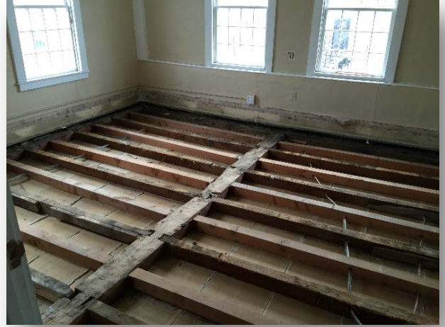
Shown Above and Below: The Loring Parsonage structural upgrades in progress.
