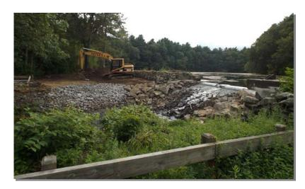
The last two pictures show the construction of a Detention Basin on the property known as 15 Hudson road adjacent to Grinnell Park. The basin is being installed to mitigate stormwater runoff from the reconstruction of Hudson Road, Concord Road and Old Sudbury Road intersection.
