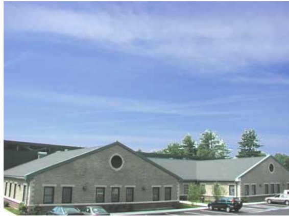
Public Works Building
