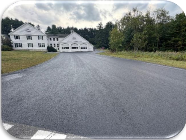
FOG SEALING PARKING LOT APPLICATION @ FIRE STATION
