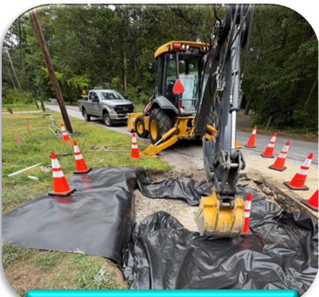
WILLOW ROAD DRAINAGE PROJECT
