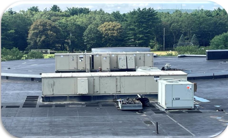
CURTIS ROOF TOP UNITS UNDER REPAIR
