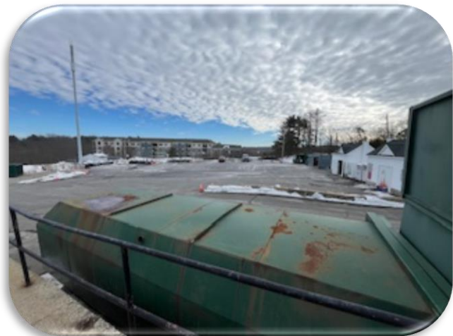
TRANSFER STATION – LOWER LOT
