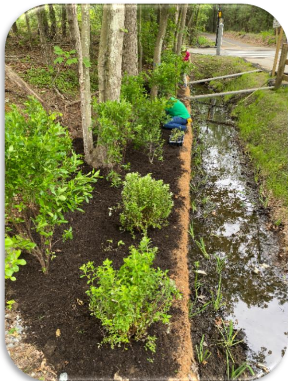
PLANTING RAIN GARDEN ON THE BRUCE FREEMAN RAIL TRAIL
