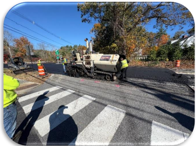
HUDSON RD @ MAYNARD ROAD PAVING
