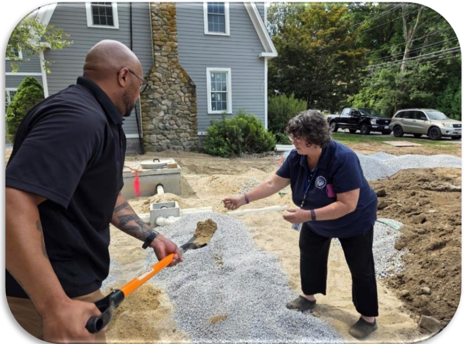
SEPTIC INSPECTION, AUGUST 14, 2025 LEFT TO RIGHT: HEALTH INSPECTOR SHAUN JEFFERY, AND REGIONAL HEALTH INSPECTOR ANN LOREE.
