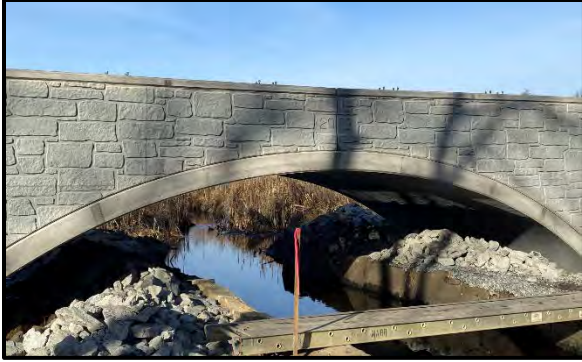
New Pantry Brook Bridge on Bruce Freeman Rail Trail
