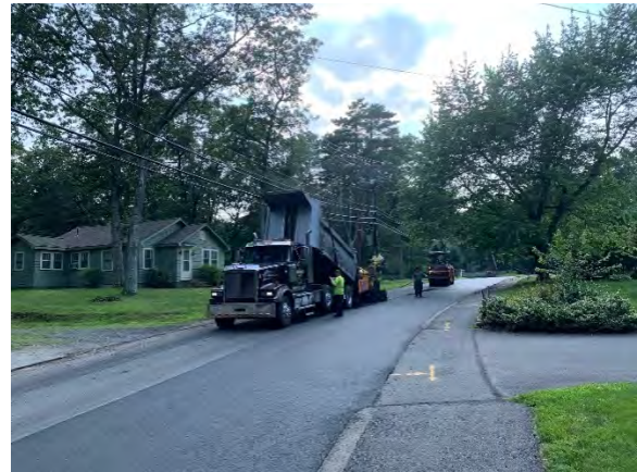
Paving of Peakham Road
