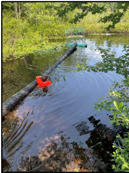
Installation of Beaver Deceiver
