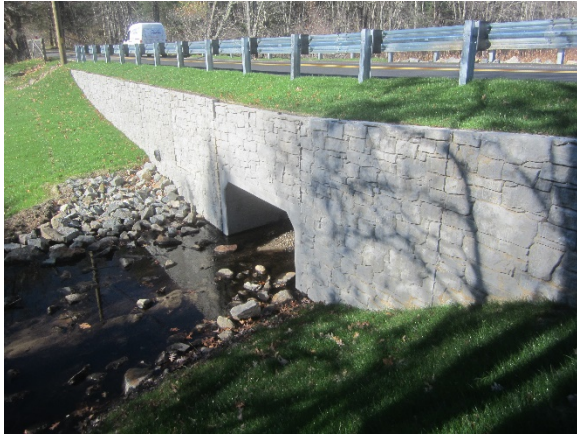
Marlboro Road Culvert Replacement Project
