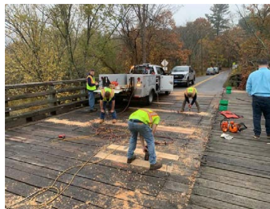
Work being completed on Sherman's Bridge.
