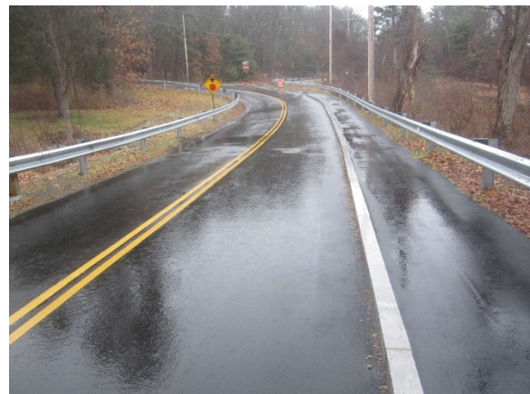
Old Framingham Road Walkway Improvement Project
