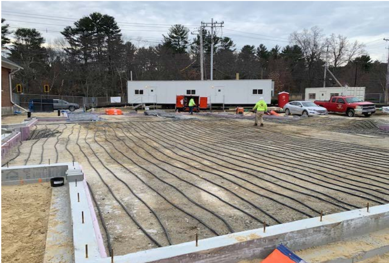
Fire Station #2 Addition Foundation, Completed December 2022
