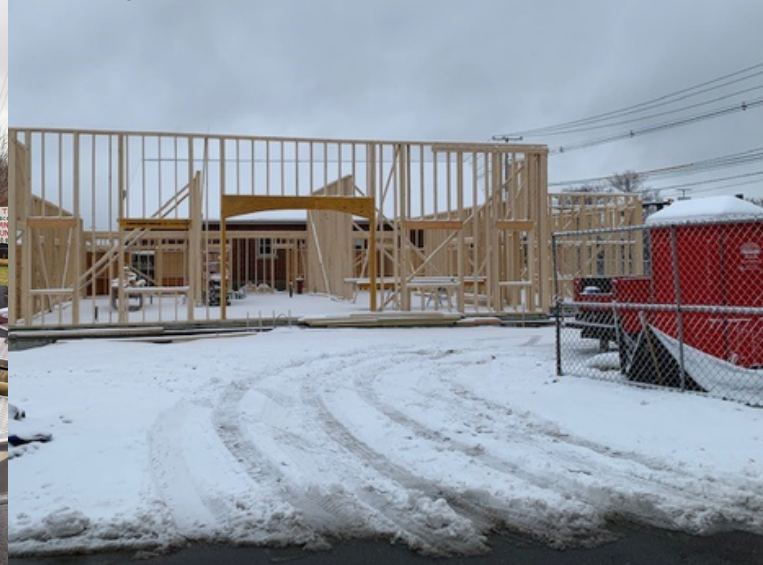
Framing the new Fire Station 2
