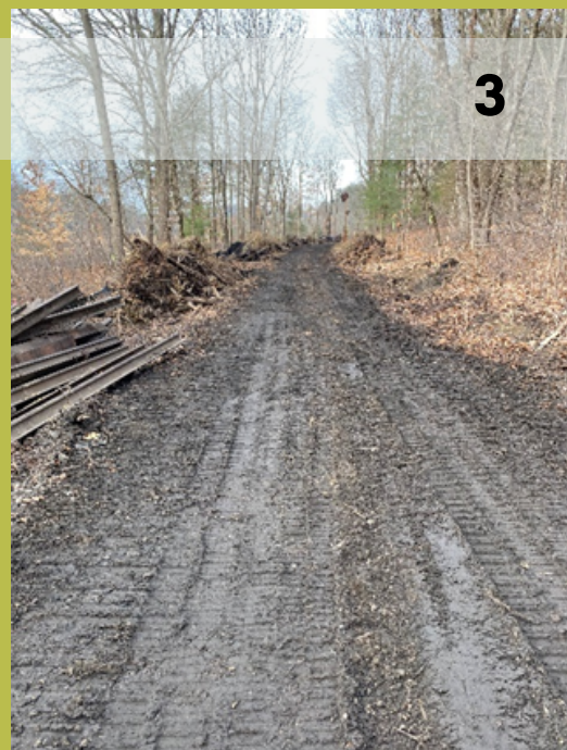
Work on the Eversource underground transmission line project shown left to right: 1) During Tree Removal, 2) Following Chipping Operation and 3) Following Rail/Tie Removal
