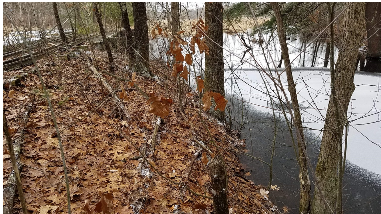
Photograph 11: Southwest side of Bridge 127. Steep slope.
