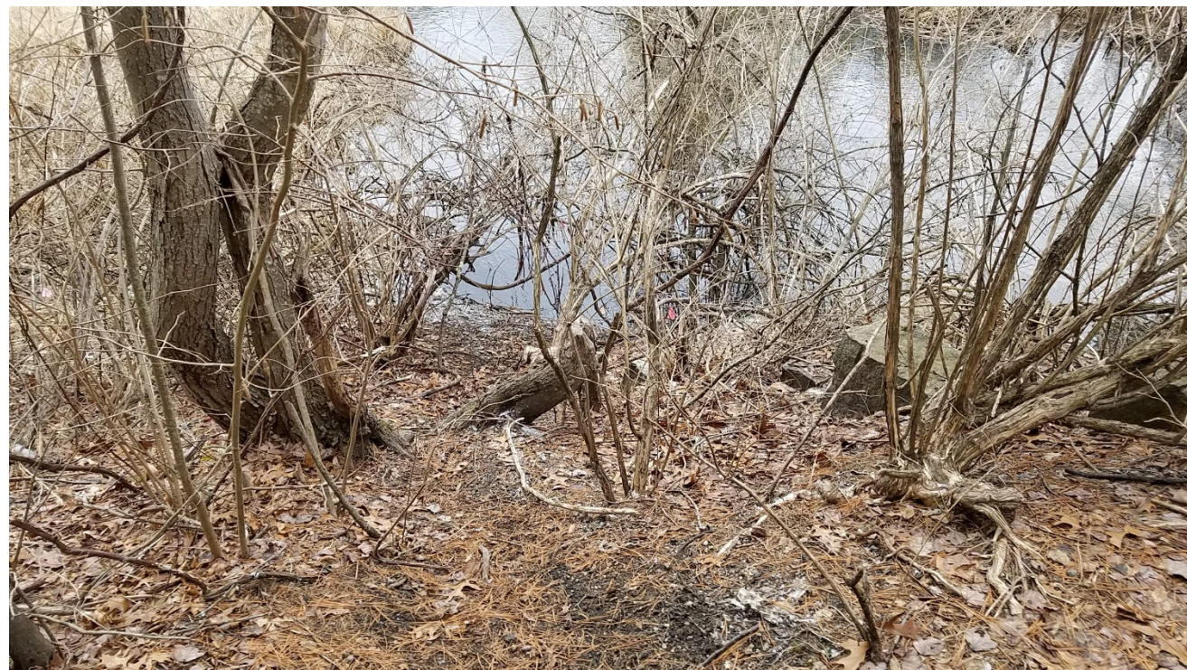
Photograph 5: Northwest side of Bridge 128. Heavily vegetated.
