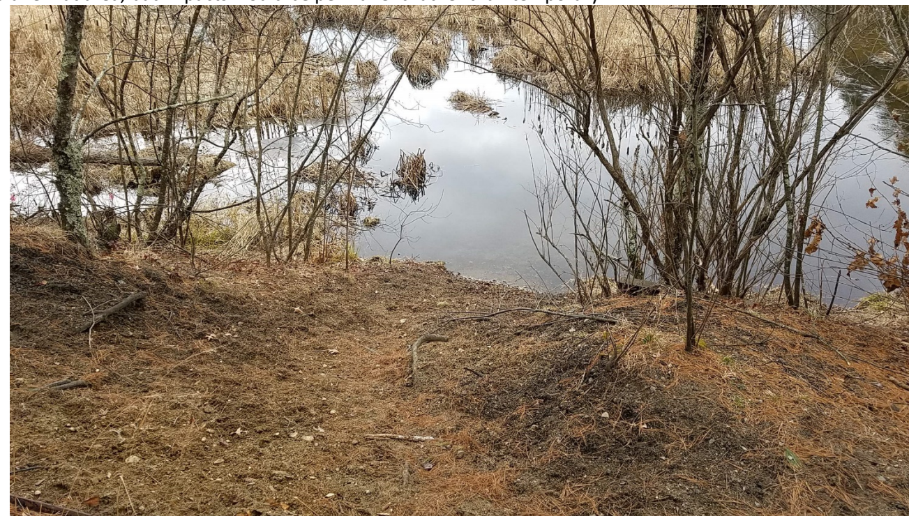
Photograph 8: Southeast side of Bridge 128. Possible but would need to confirm if water depth is sufficient.
