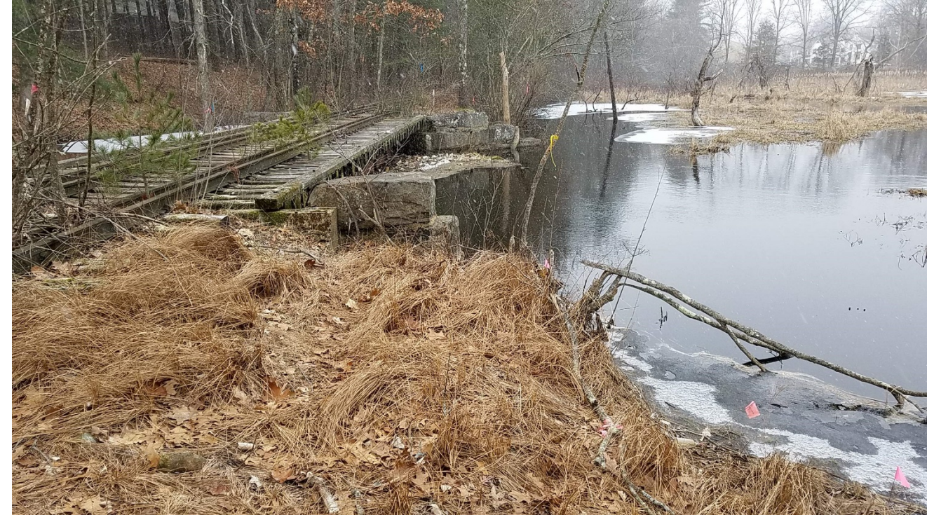
Photograph 10: Northeast side of Bridge 127. Gentle slope.
