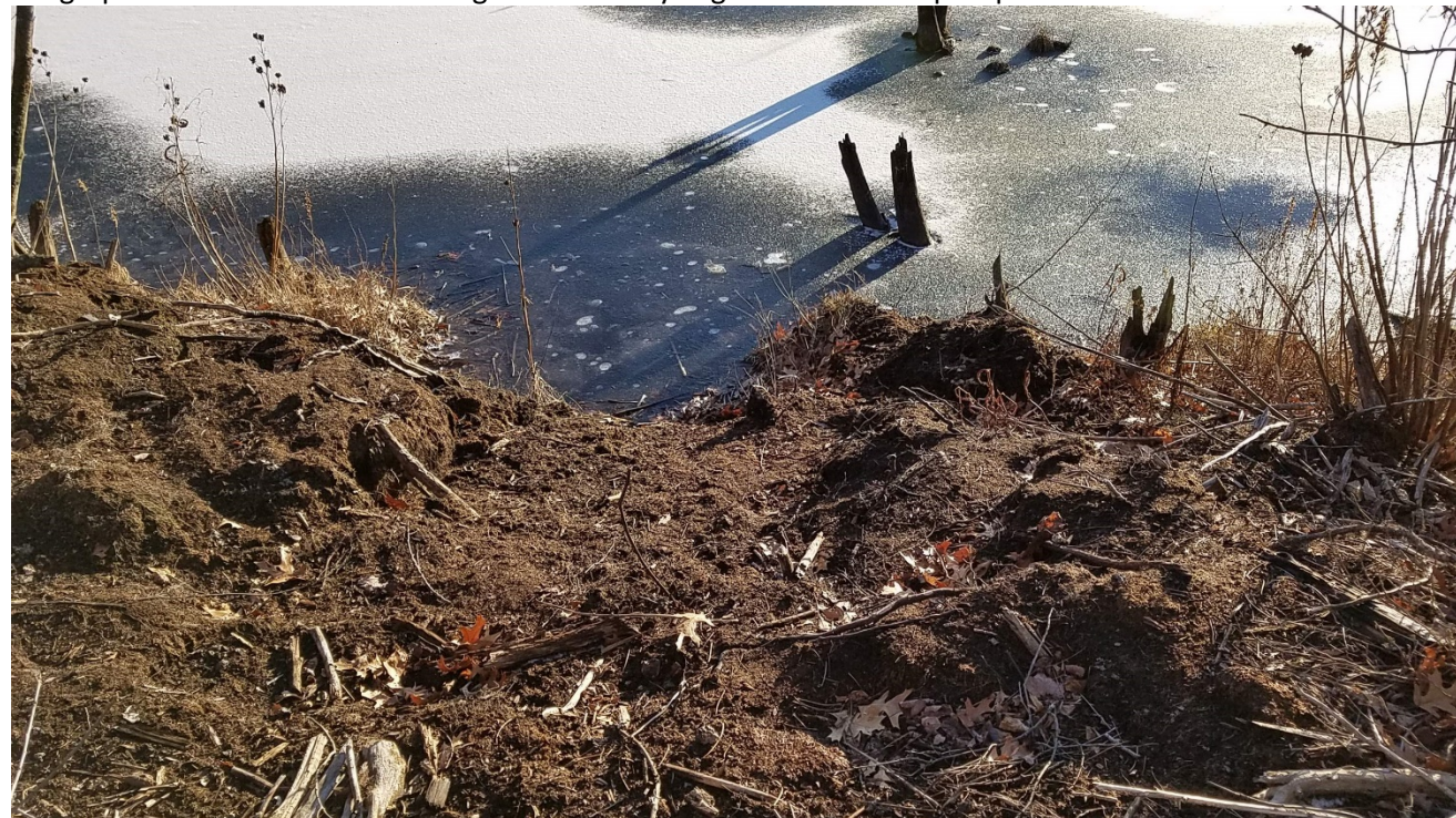
Photograph 3: Southwest side of Bridge 130. Steep slope.
