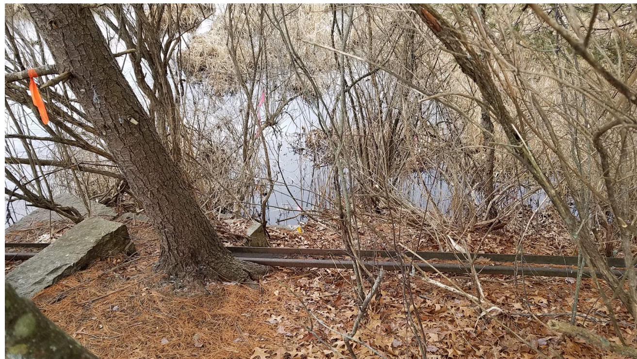
Photograph 7: Southwest side of Bridge 128. Heavily vegetated.
