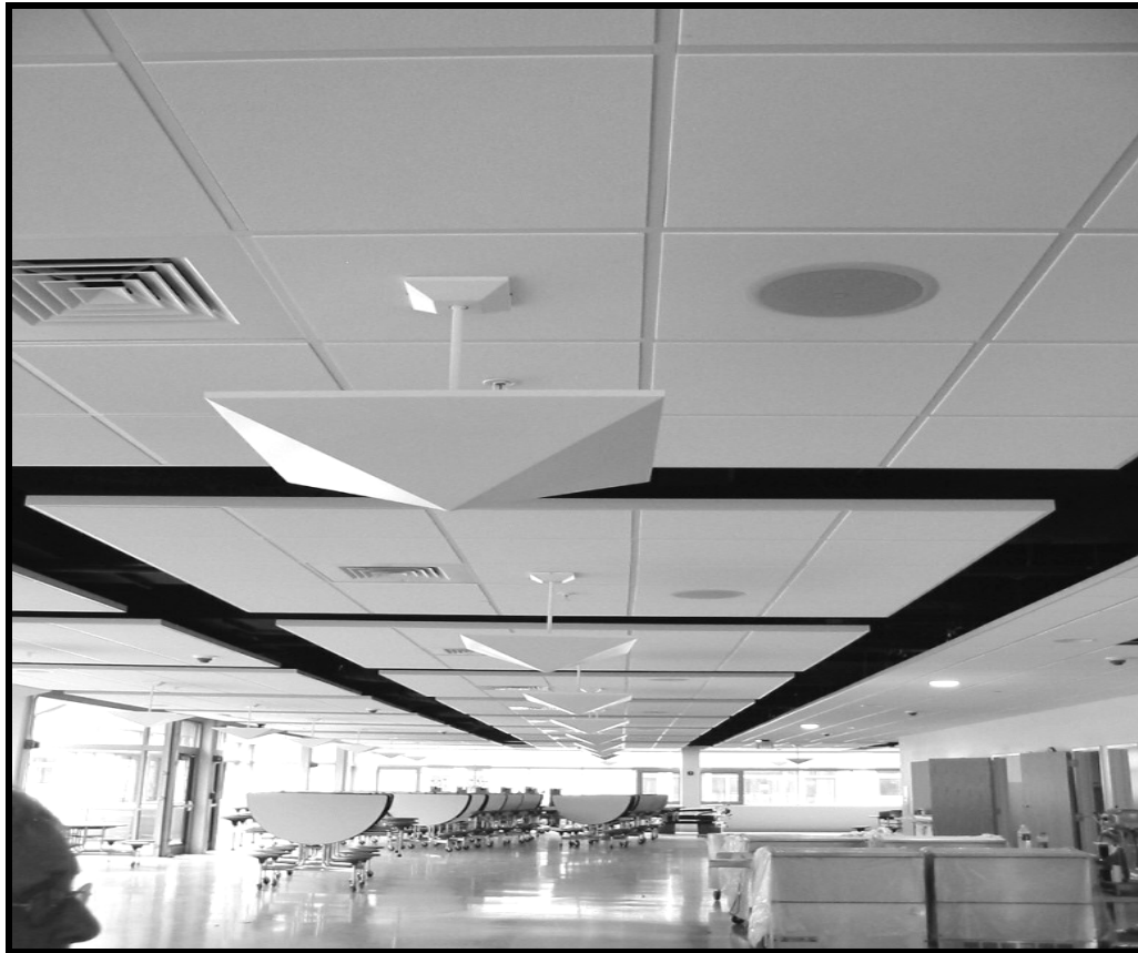
The new Cafeteria Commons at LSRHS. (Photo Courtesy of Timothy Coyne)
