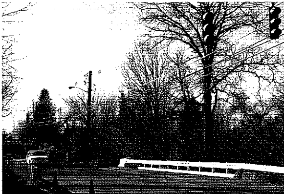
Landham Road Bridge construction Photo: Joe Skinnion
