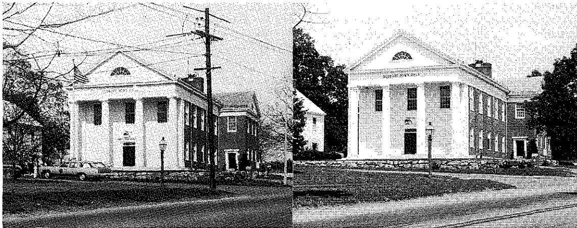
BEFORE AND AFTER: SUDBURY CENTER with and without power lines. The juice now flows underground (Carl Alsen photo).
