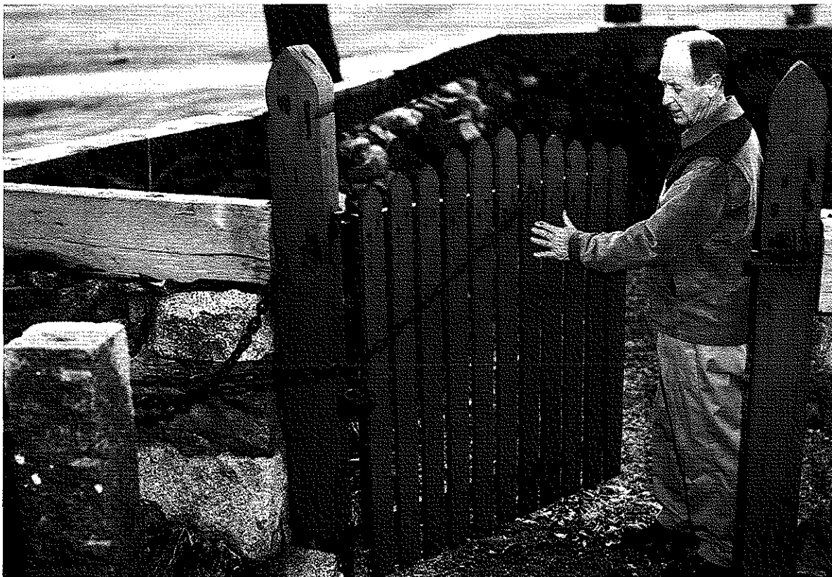
AT LAST, AFTER MANY DECADES, Sudbury's animal pound has a door, thanks to Pound Keeper Sam Reed, its builder, who demonstrates his ingenious self-closing arrangement whereby the weight on the chain pulls the door closed when released. (Clay Allen photo)
