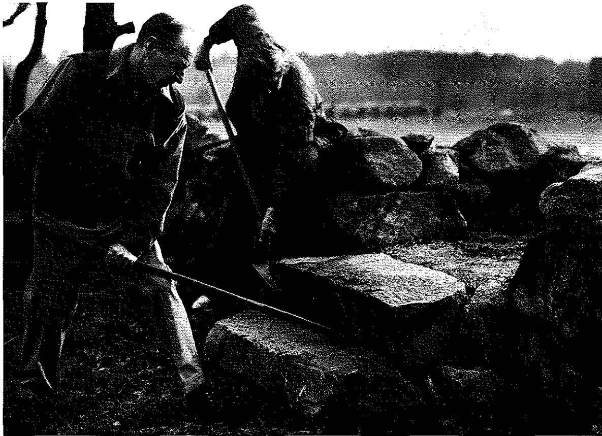
SETTING THE LAST STONE in place, Sam Reed, left, and Dick Gustafson thereby complete the passageway thru the stone wall between the Town Hall parking lot and the Revolutionary War cemetery. Sam and Dick spent many hours during the past year rebuilding the entire wall around the cemetery.
