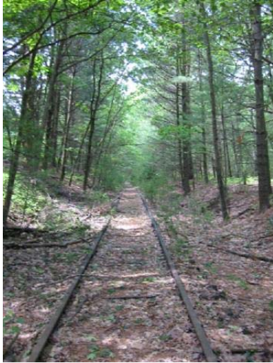
Figure 14: Minimal Vegetative Growth
