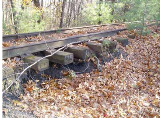
Figure 23: Existing Eroded Area
