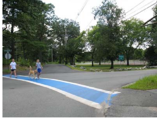
Figure 54: Existing Crosswalk at Concord Road / Morse Road
