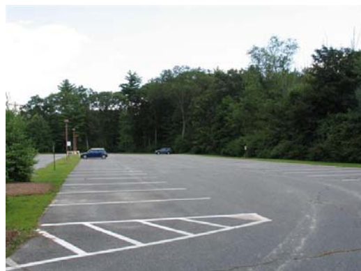
Figure 53: Nixon Elementary School Parking Lot
