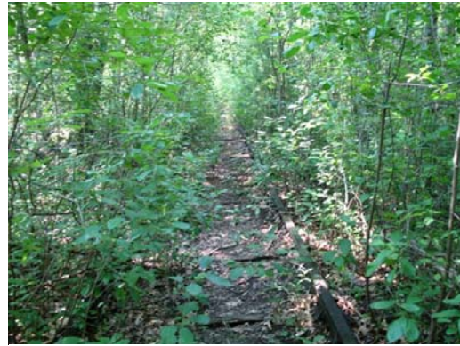
Figure 15: Substantial Vegetative Growth
