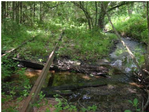
Figure 16: Washed Out Culvert at Stream Crossing
