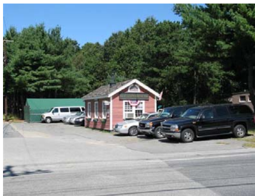
Figure 8: Existing Railroad Station Building
