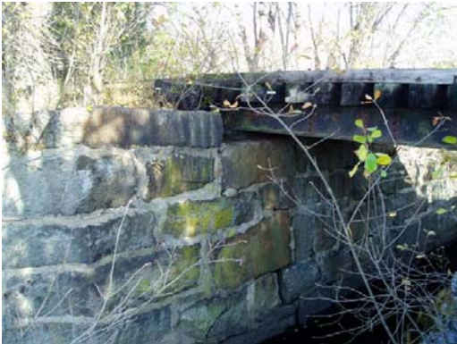
Figure 36: Pantry Brook Trestle
