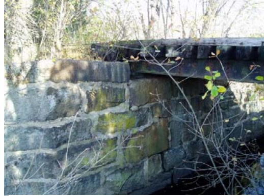
Figure 5: Pantry Brook Railroad Trestle
