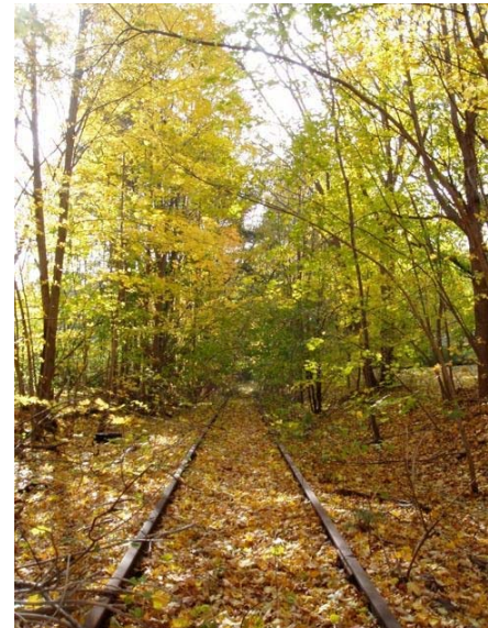
Figure 3: Railbed South of Hudson Road (Route 27)
