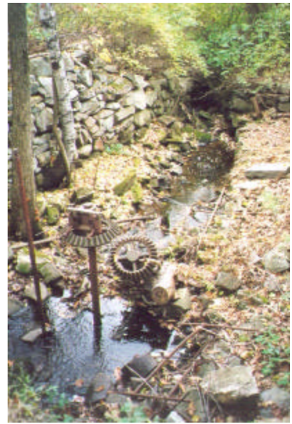
Figure 47: Old Stone Mill Foundation - Pencil Factory Dam Site
