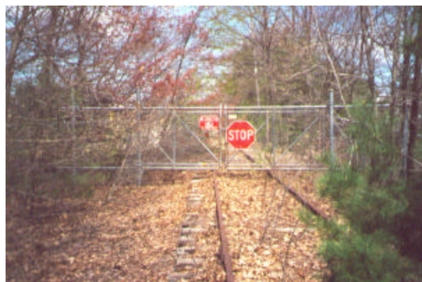
Figure 12: Rex Lumber Encroachment Fencing Across the Right-of-Way
