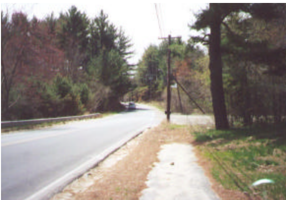
Figure 31: Route 27 Looking South
