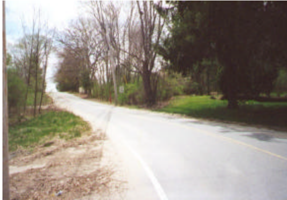
Figure 21: Wetherbee Street Looking West
