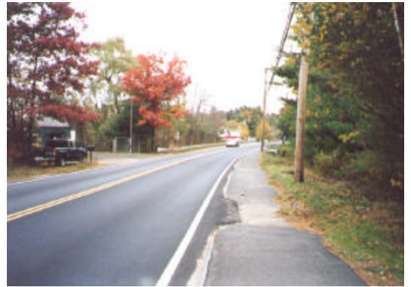
Figure 30: Route 27 at Ledge Rock Way - Looking North
