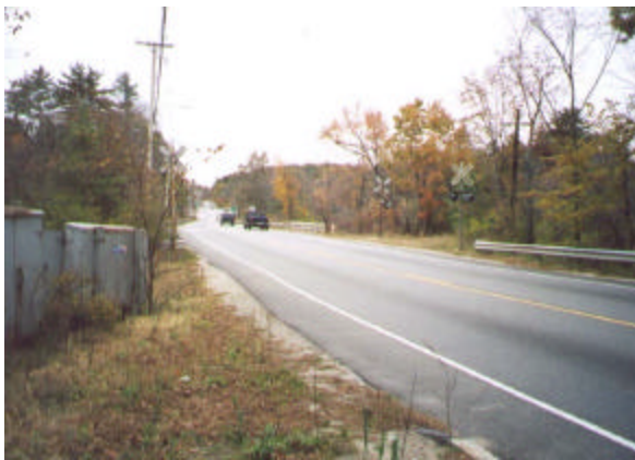
Figure 27: Great Road (Route 2A/119) Looking West
