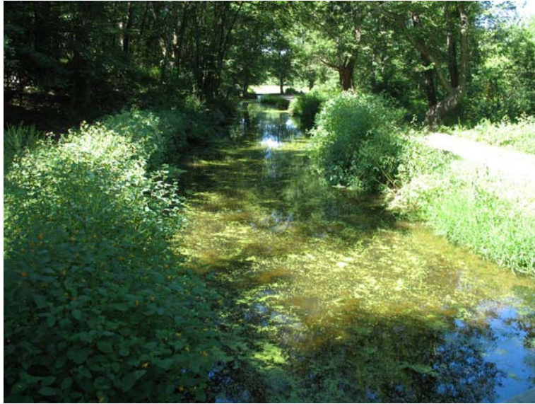
Figure 6: Sluiceway looking toward dam
