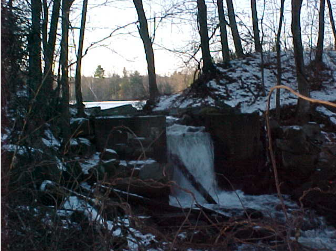
View of Hager Pond and Hager Pond Dam, Marlborough, MA
