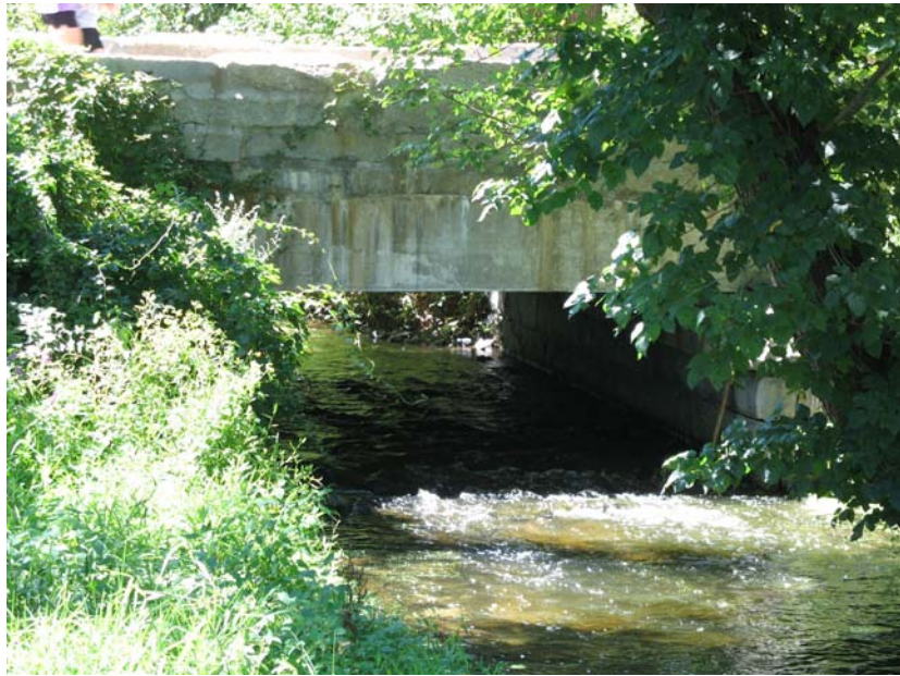
Figure 10(a): Culvert under Wayside Inn Road
