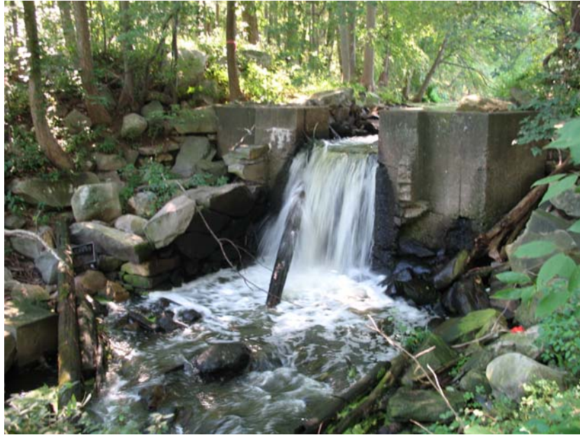
Figure 2: Weir Structure at Hager Pond Dam – Upstream View
