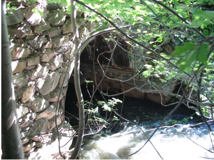
Figure 5: Culvert under Hager Street downstream of Hager Pond Dam
