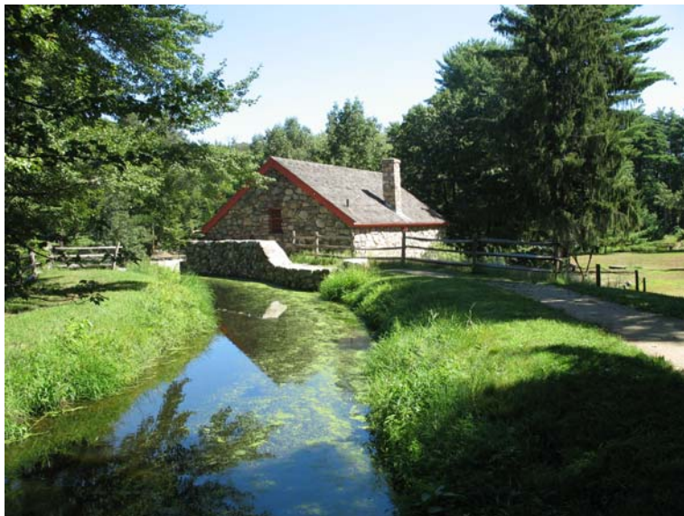
Figure 7: Sluiceway looking toward Grist Mill
