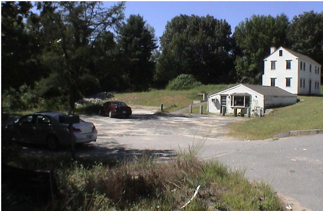
Figure 10: Recommend Dewatering Site – Evie's Attic Antiques
