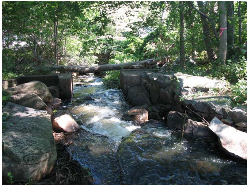
Figure 3: Weir Structure at Hager Pond Dam – Downstream View
