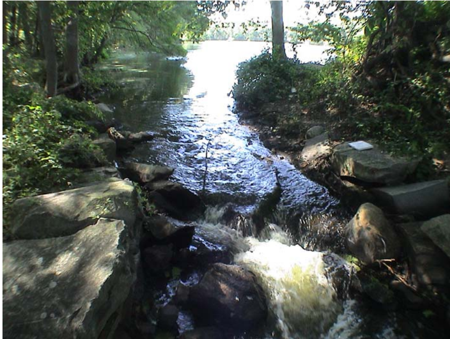
Figure 4: Inlet to Hager Pond Dam
