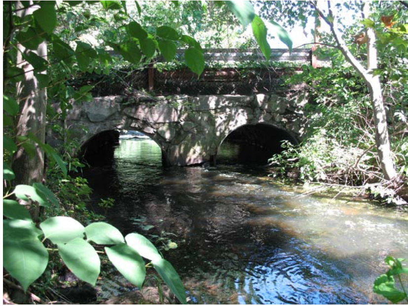
Figure 6: Culvert under Dutton Road
