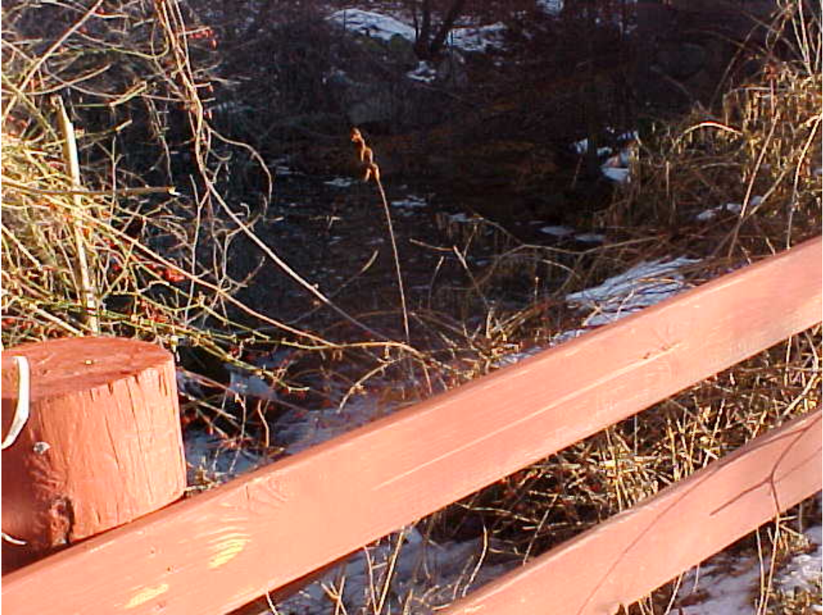
Looking easterly while standing on bridge, Carding Millpond Dam
