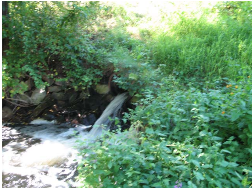
Figure 5: Outlet pipe at Toe of Earth Dam
