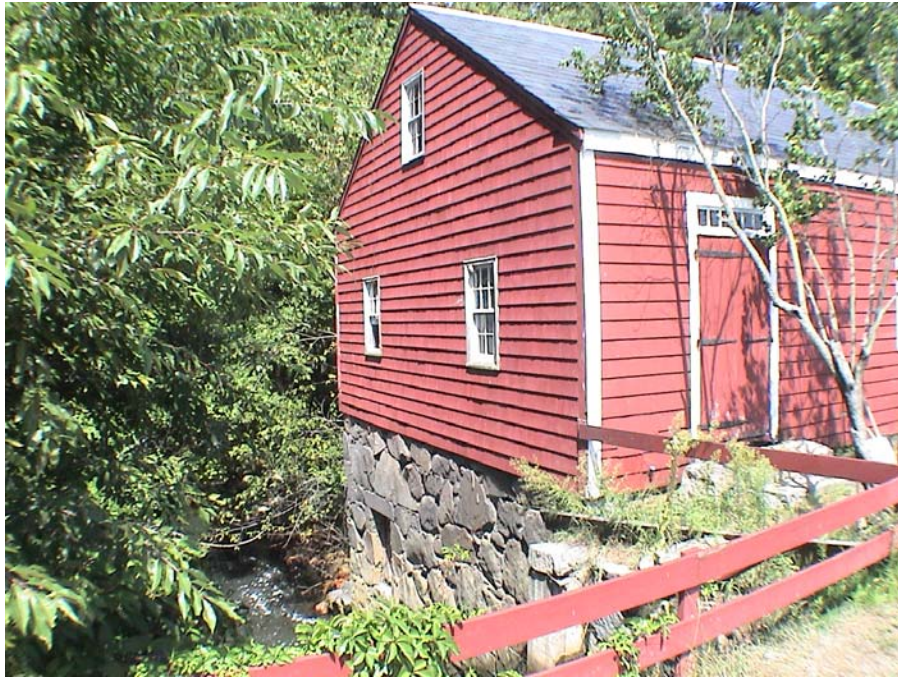
Figure 2: Carding Millpond Building Adjacent to Spillway (Note: Orange staining beyond rock foundation)
