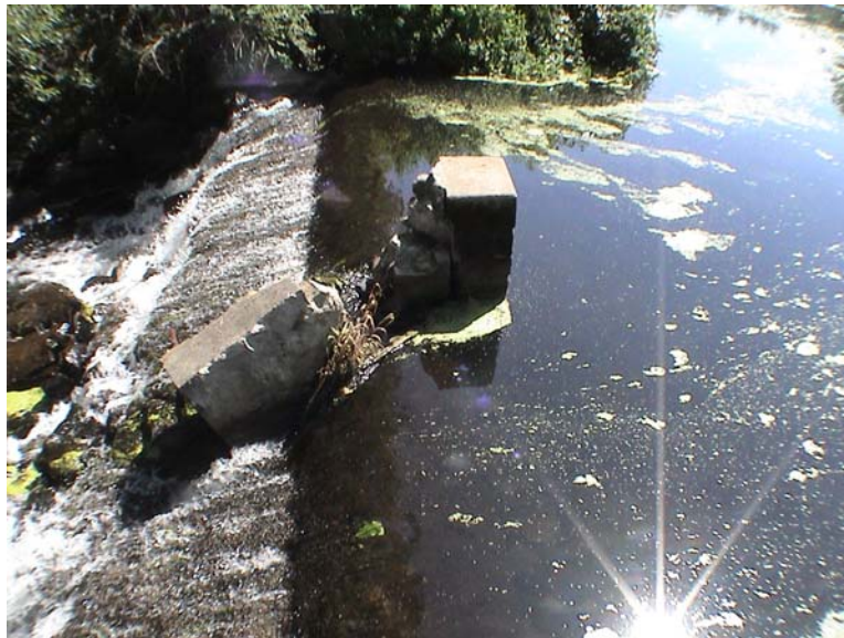
Figure 5: Concrete Spillway Section
