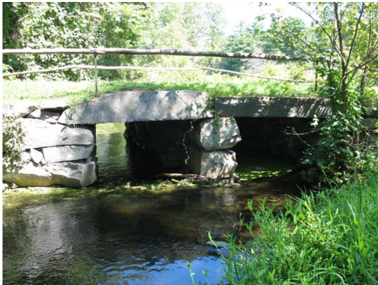
Figure 10(b): Stone Culvert under Service Road to Wayside Inn
