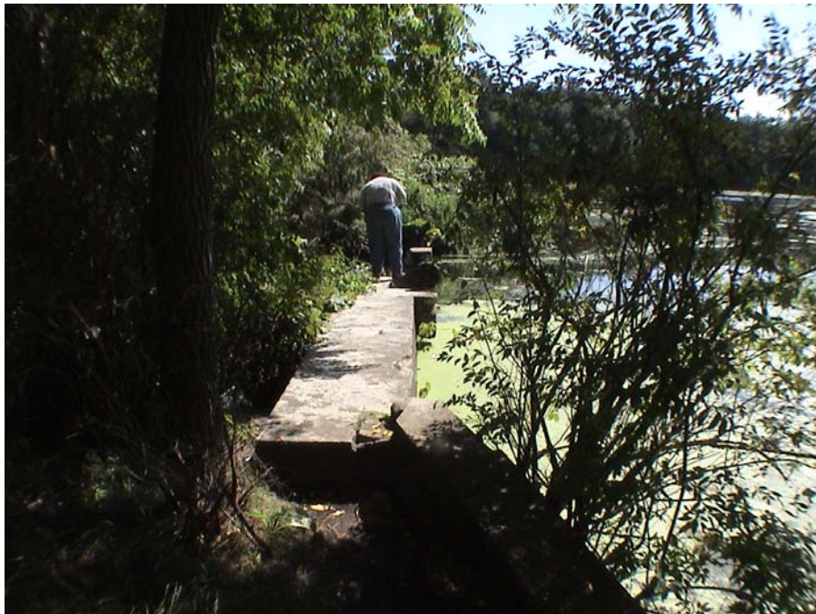
Figure 3: Concrete Walls on Left Abutment
