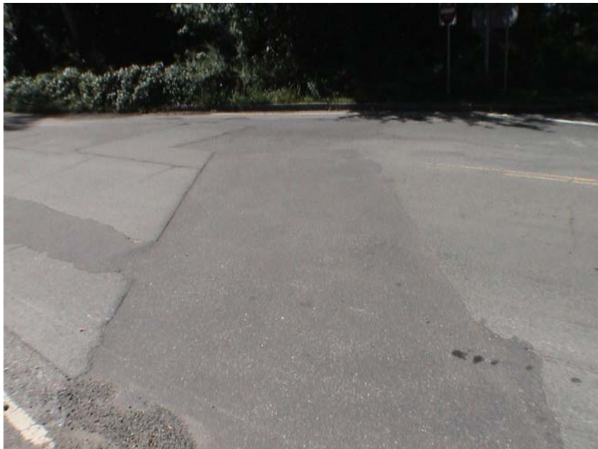
Figure 6: Repairs to Culvert under Hager Street (looking toward Hager Dam)
