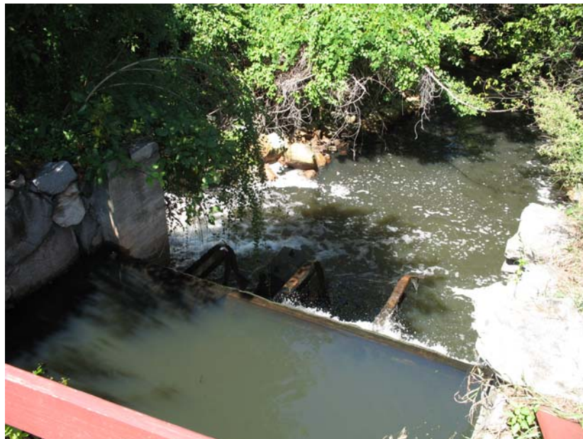
Figure 5: Stop Logs – Controlled Spillway
