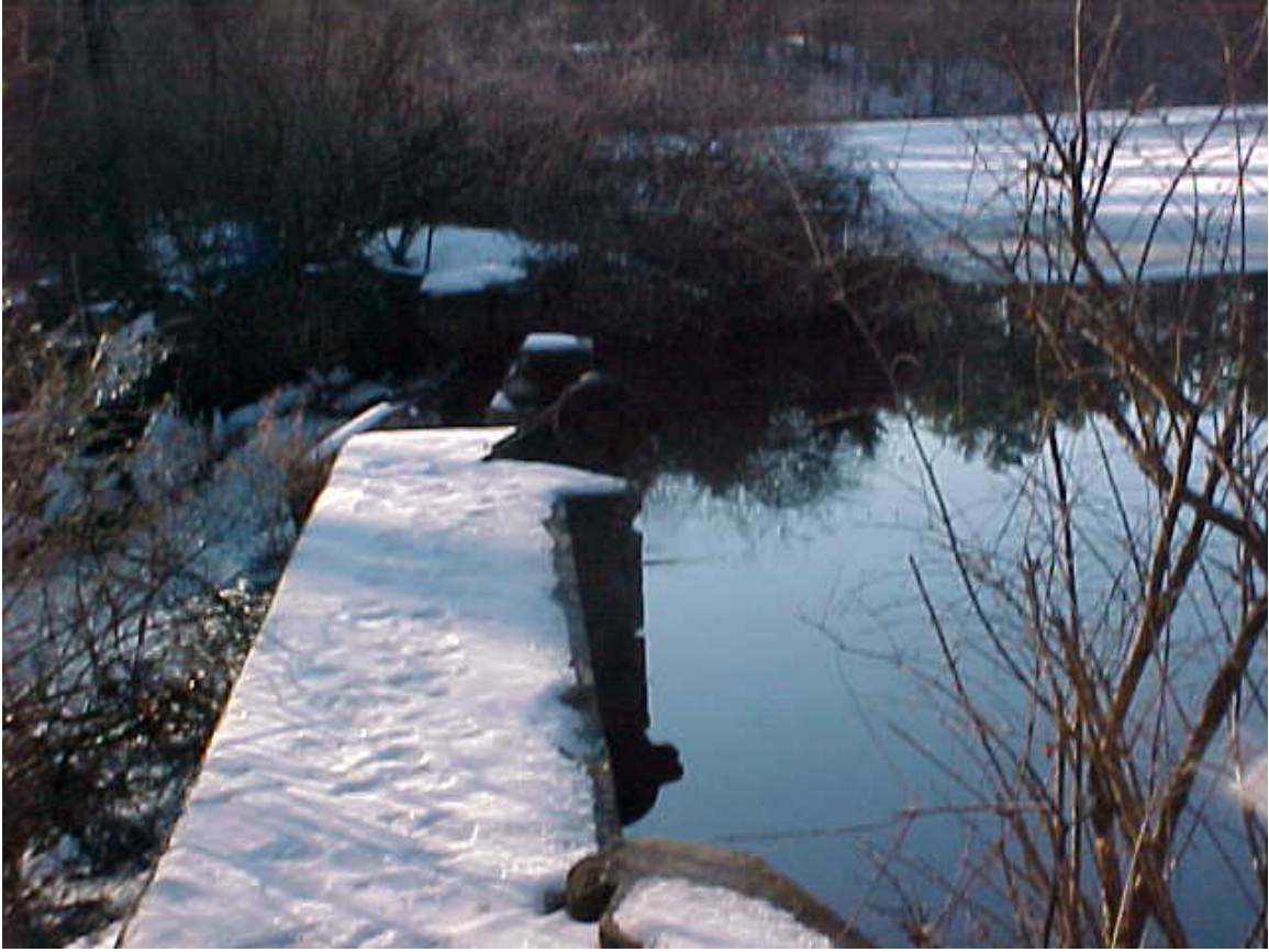
Stearns Millpond Dam, off Dutton Road, Sudbury, MA
