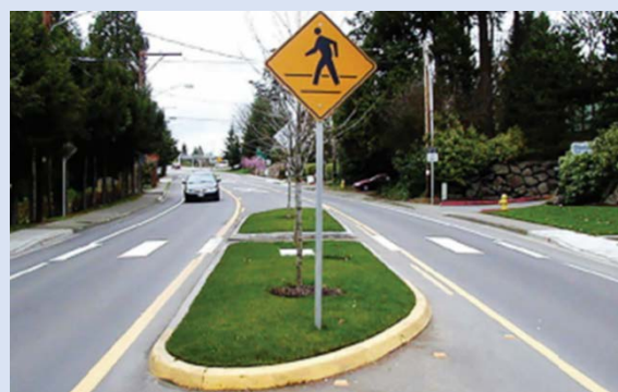
Example median and pedestrian refuge island
