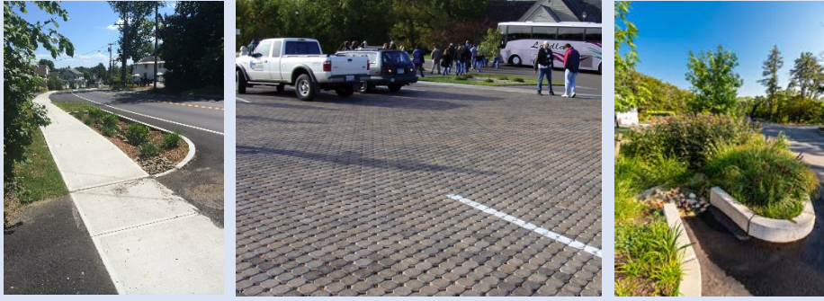
Green infrastructure and low impact design include the use of rain gardens and plantings (left and right) and pervious pavers (center) to manage stormwater.
