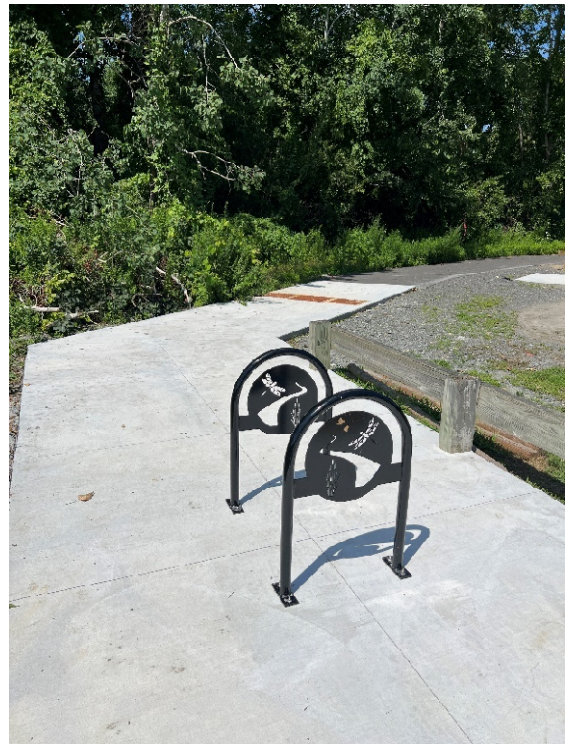
Photo 20: Sta. 1108+00 looking at the concrete work and new bicycle racks.
