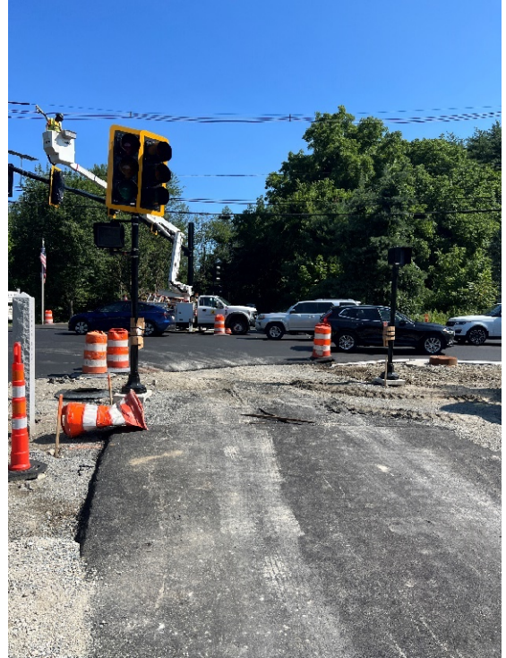
Photo 10: Looking at the proposed traffic signal posts and signal heads.
