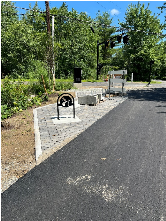
Photo 17: Sta. 306+50 looking at the rest area south of North Road.
