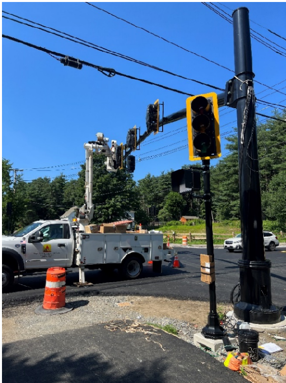
Photo 11: Looking at the installation of conduit through the mast arm.
