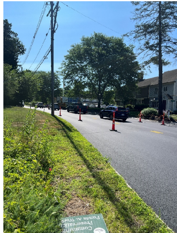
Photo 8: Looking at the milled and overlaid section of Hudson Road.
