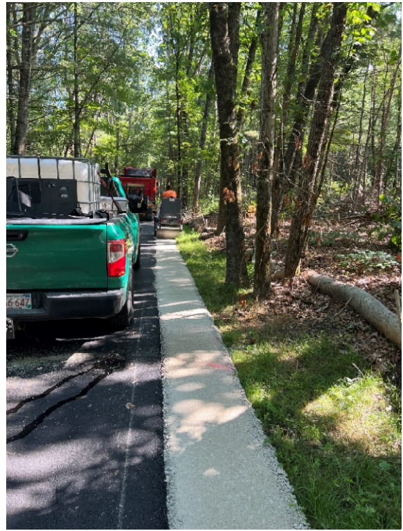
Photo 6: The crushed stone shoulder being graded.
