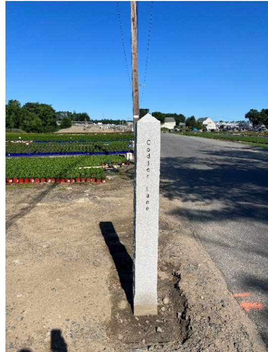
Photo 2: Sta. 116+00 looking at the granite pier for the Codjer Lane crossing.
