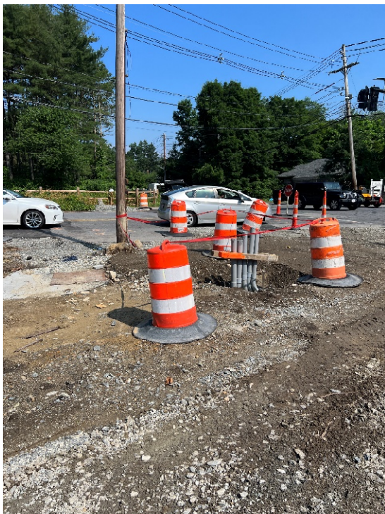
Photo 7: Looking at the location of the proposed traffic controller.
