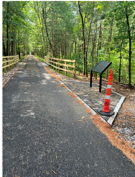
Photo 16: Sta. 259+00 looking at the pervious paver rest area and interpretive sign.
