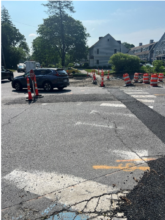
Photo 9: Looking at the pavement patching where the previous island used to be in Peakham Road.
