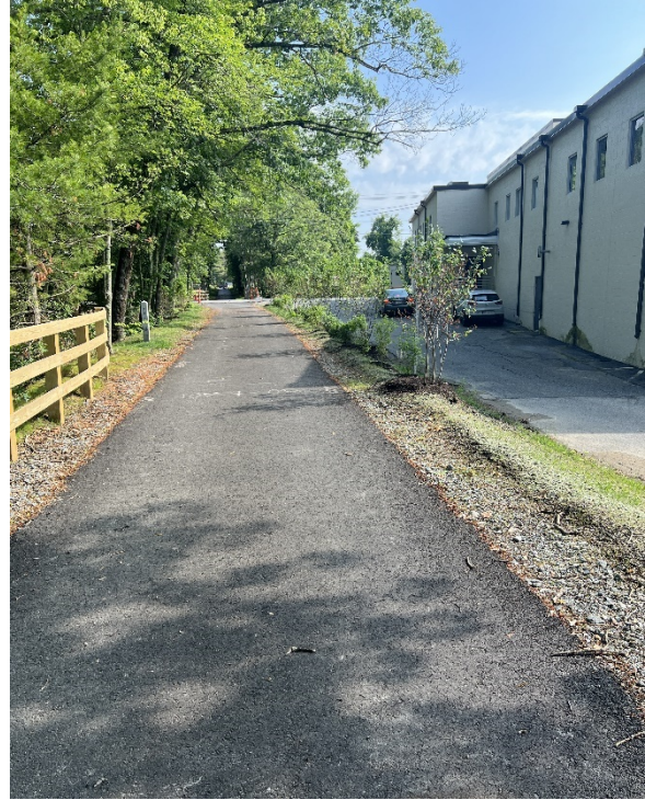
Photo 2: Sta. 106+50 looking at the plantings south of the 71 Union Driveway.
