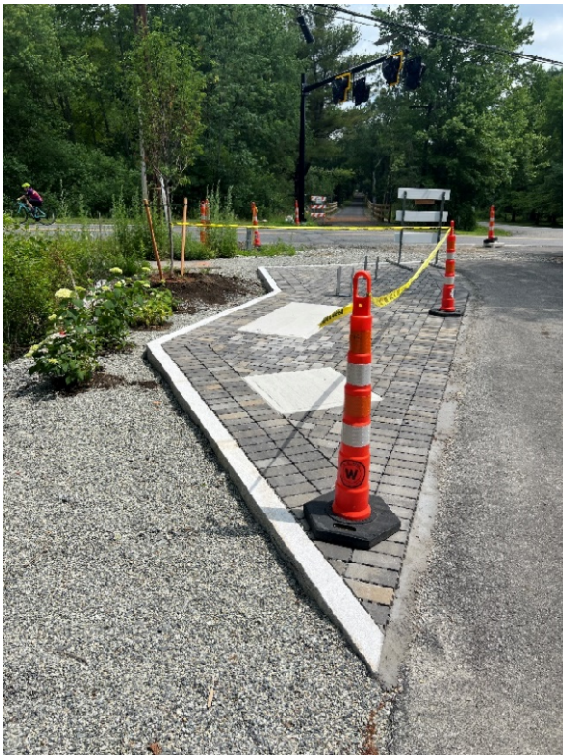
Photo 19: Sta. 306+50 looking at the rest area south of North Road.
