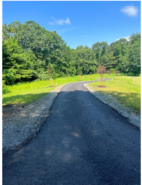
Photo 10: Sta. 184+50 looking at the plantings along the Parkinsons Lot Spur Path.
