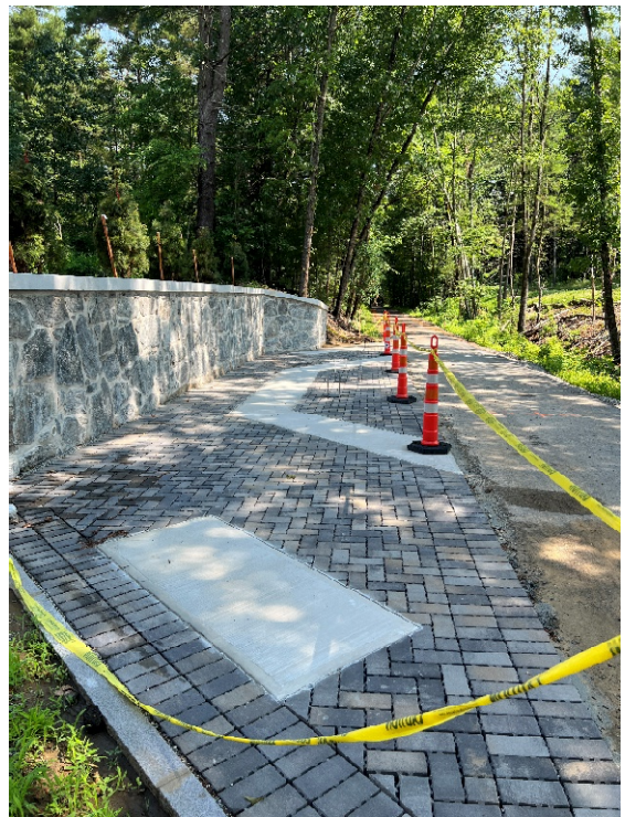
Photo 12: Sta. 216+50 looking at the rest area north of Morse Road.
