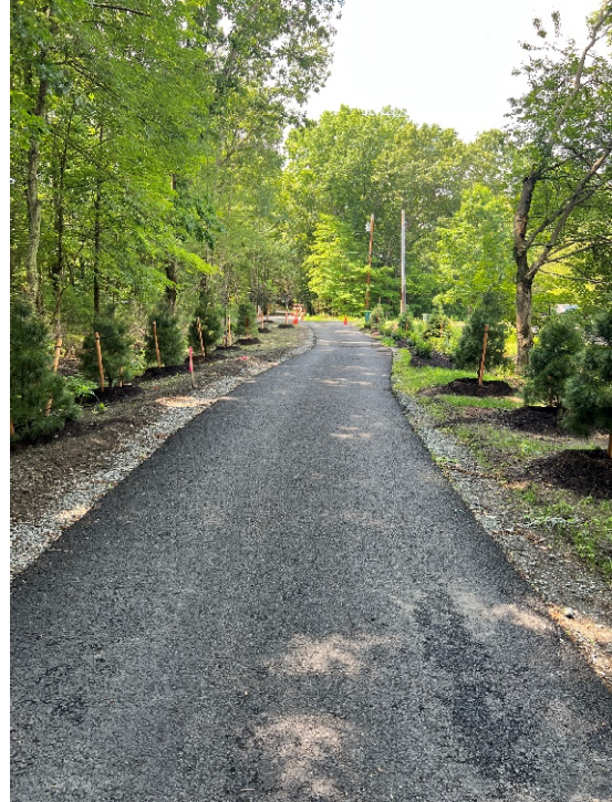
Photo 18: Sta. 277+00 looking towards Haynes Road at the plantings.
