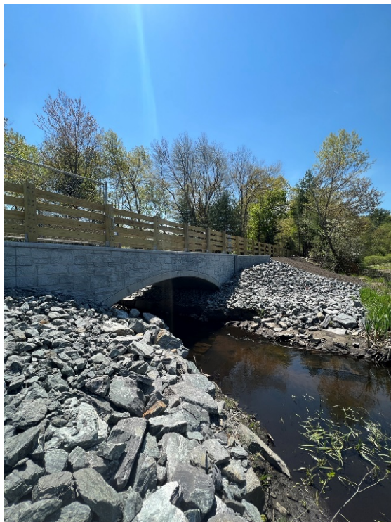
Photo 11: Sta. 265+00 looking at the constructed bridge over Pantry Brook.
