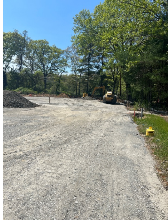
Photo 4: Progress photo of the parking lot grading at Morse Road.
