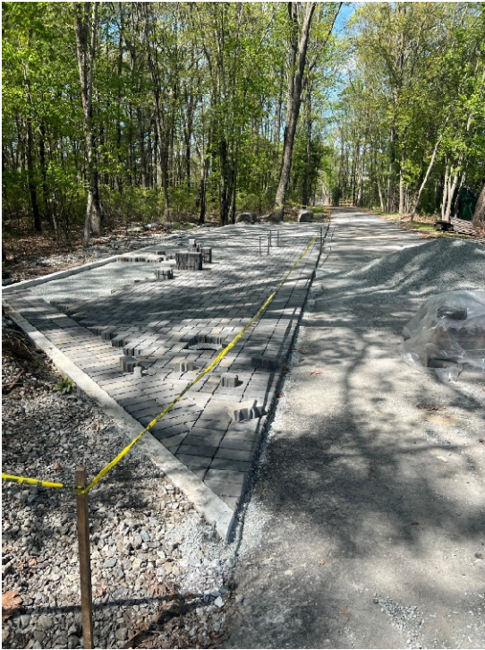
Photo 1: Sta. 101+00 looking at the rest area at the beginning of the project.
