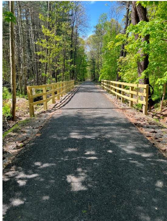
Photo 8: Sta. 168+00 looking south at the 48-inch culvert and fencing.
