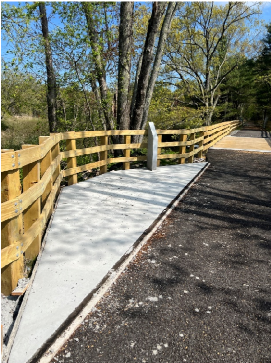
Photo 7: Sta. 125+50 looking towards Hop Brook and the proposed rest area.
