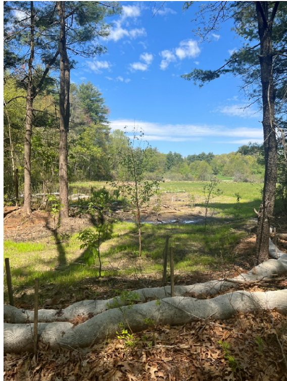
Photo 10: Sta. 213+00 looking at the wetland replication area south of Morse Road.
