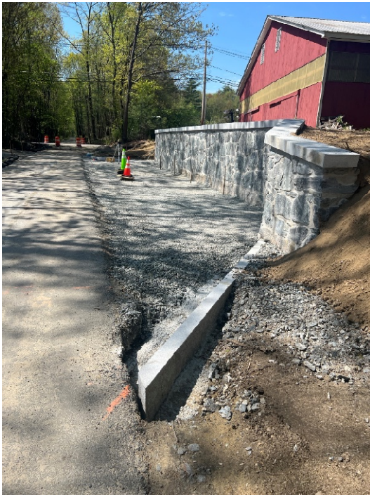
Photo 3: Sta. 217+50 looking south towards the retaining wall and Morse Road.
