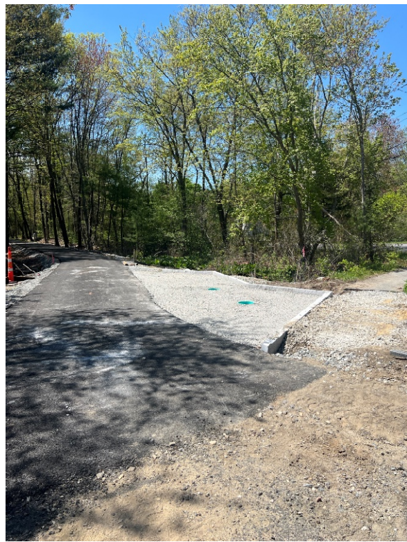
Photo 6: Sta 307+50 looking south at the rest area south of North Road.
