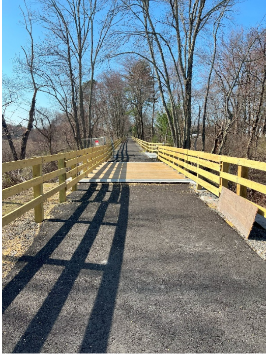
Photo 1: The completed fencing over Hop Brook.
