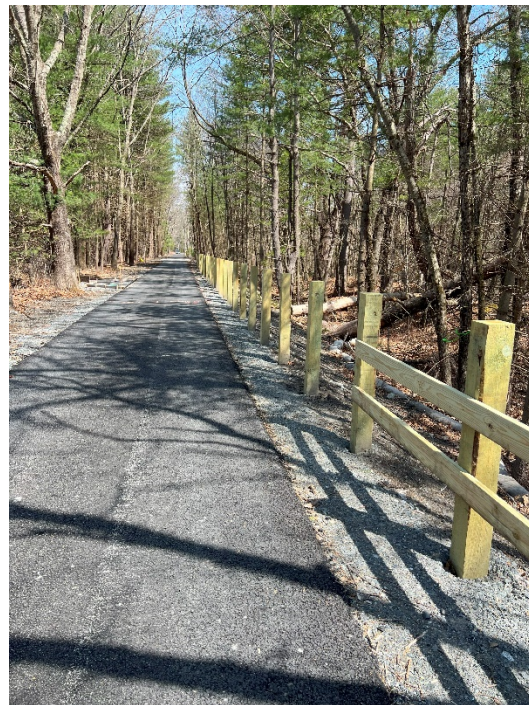
Photo 8: Sta. 267+00 looking north at fence installation progress.
