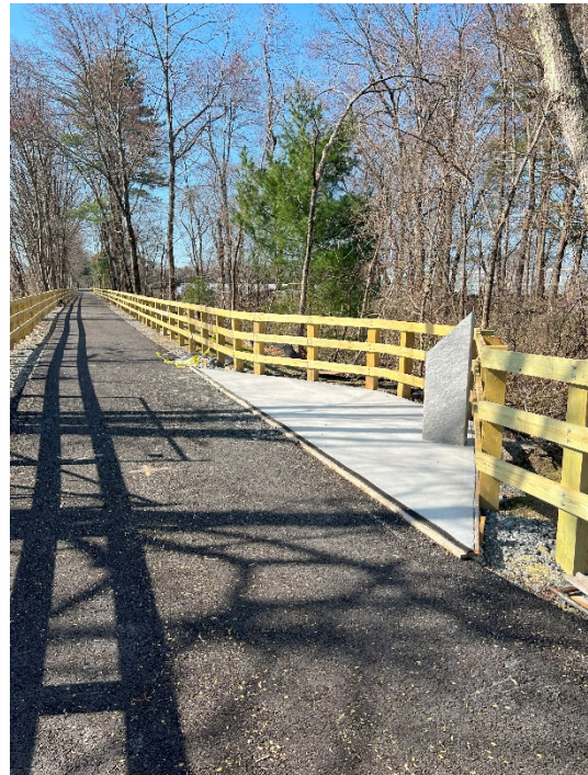
Photo 2: Sta. 126+50 looking south at the concrete rest area.
