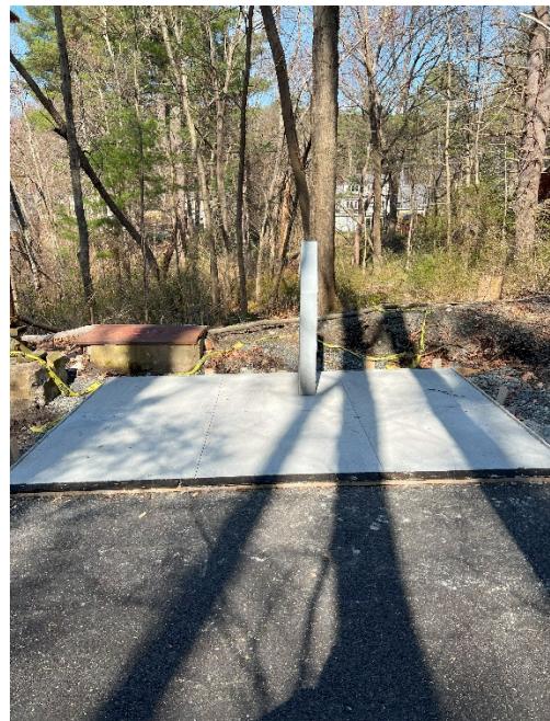
Photo 4: Sta. 163+00 looking at the concrete rest area.
