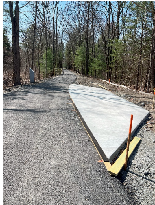
Photo 10: Sta. 275+00 looking at the rest area south of Haynes Road.
