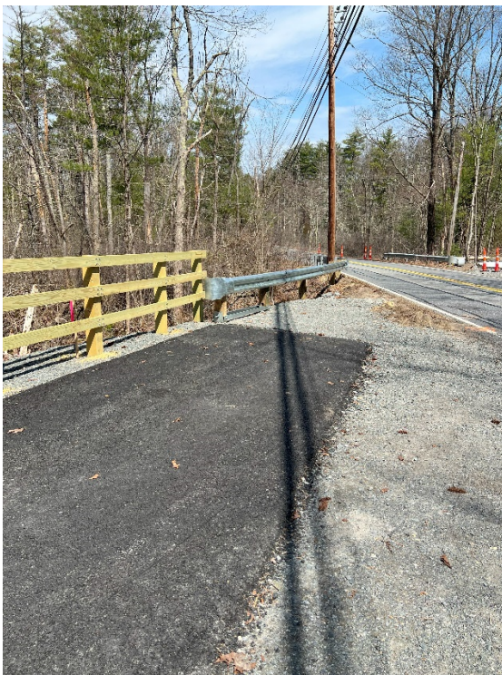
Photo 11: Sta. 284+00 looking at the constructed fencing and guardrail.
