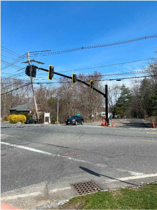
Photo 5: Sta 175+00 looking at the constructed traffic signal over Hudson Road.
