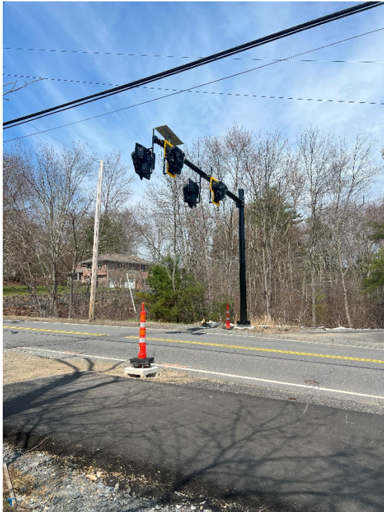
Photo 13: Sta. 307+50 looking at the HAWK signal above North Road.
