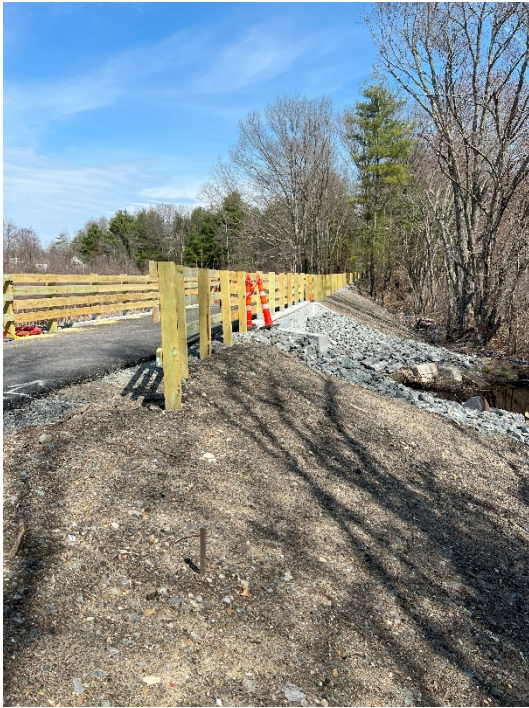
Photo 9: Sta. 264+00 looking at the fencing across the Pantry Brook bridge.
