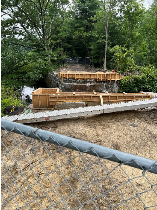
Photo 1: Sta. 127+00 looking south at Hop Brook
