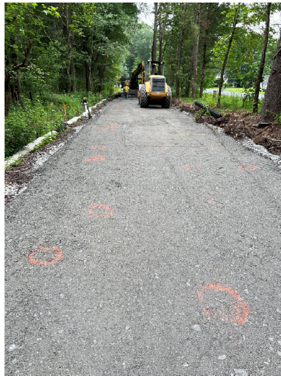
Photo 8: Sta. 281+00 looking south at new gravel being placed and graded
