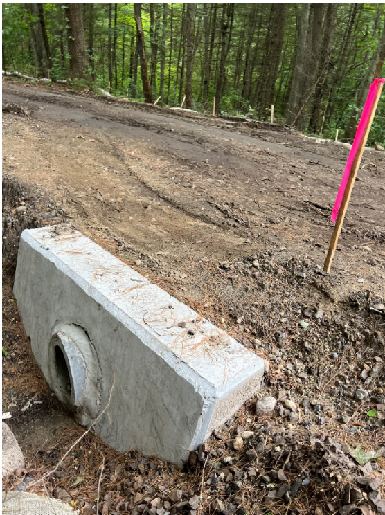
Photo 7: Sta. 283+50 looking at new headwall near Pantry Road
