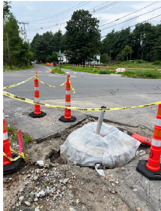
Photo 2: Sta. 176+00 looking at new signal mast foundation at Hudson Road.
