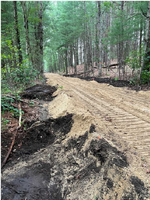
Photo 5: Sta 252+00 looking north at freshly placed fill material
