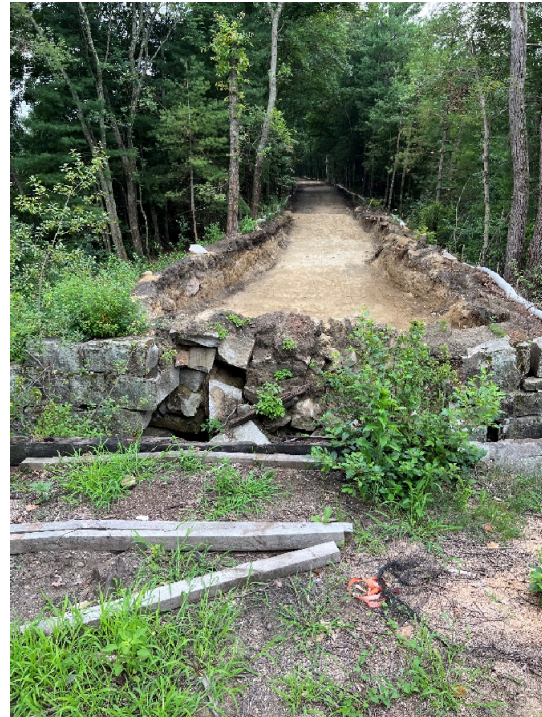
Photo 6: Sta. 265+00 looking south at excavation around Pantry Brook
