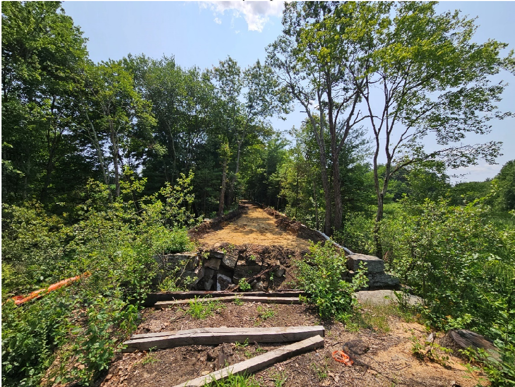
Photo 10. Pantry Brook Bridge looking south.
