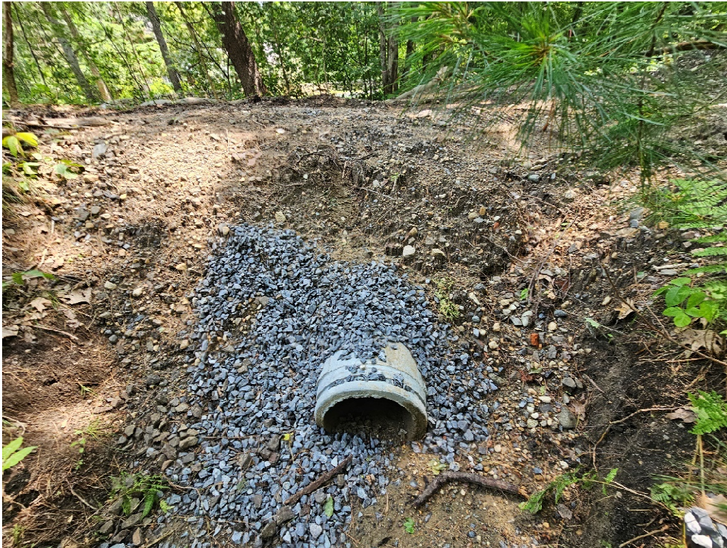
Photo 13: RFI #001: 12" RCP & headwall installed south of Pantry Road
