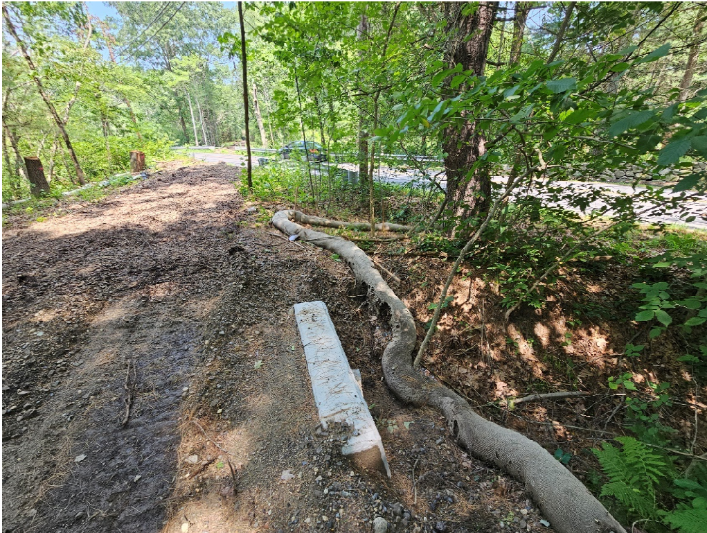
Photo 11. RFI #001: 12" RCP & headwall installed south of Pantry Road
