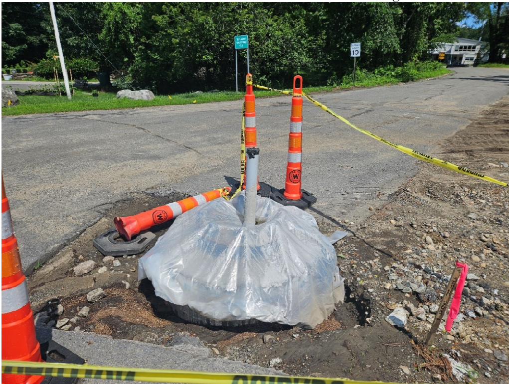
Photo 4 Mast Arm foundation at Ti-Sales
