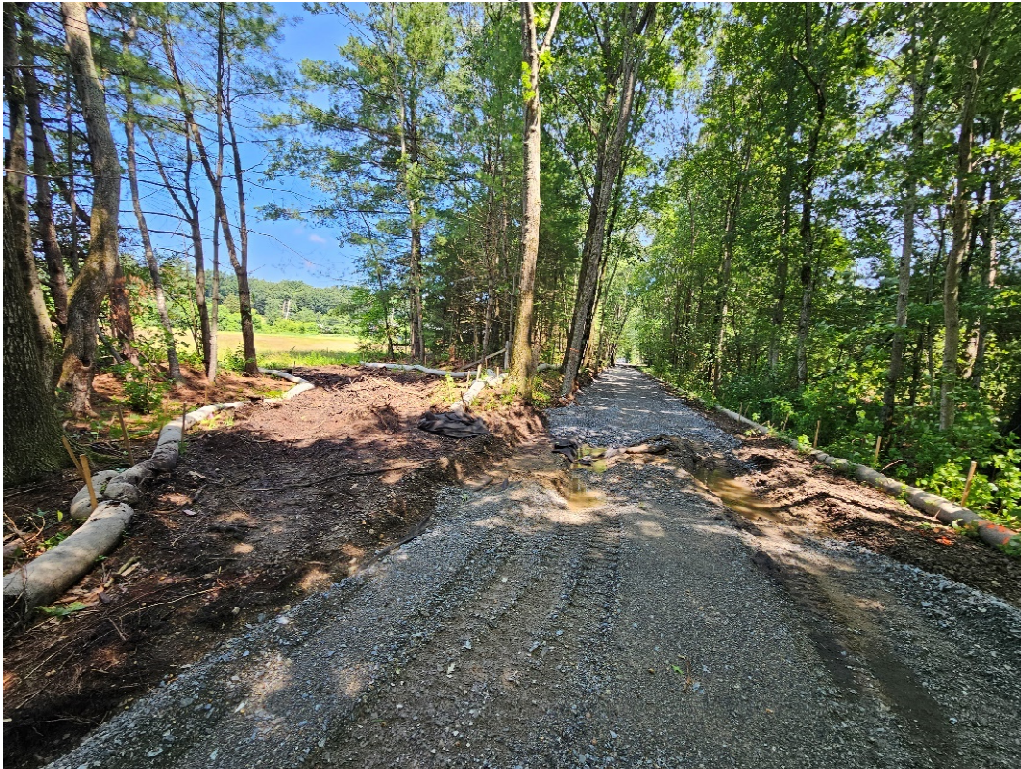
Photo 8. Excavation and entrance to wetland replication area.
