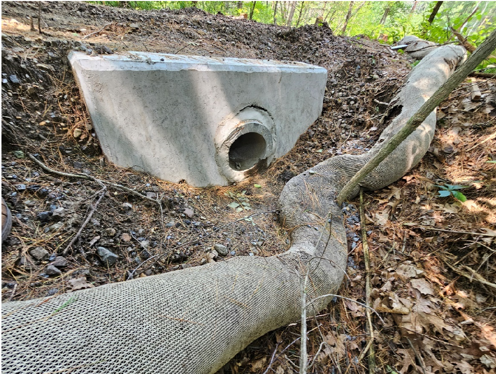
Photo 12. RFI #001: 12" RCP & headwall installed south of Pantry Road
