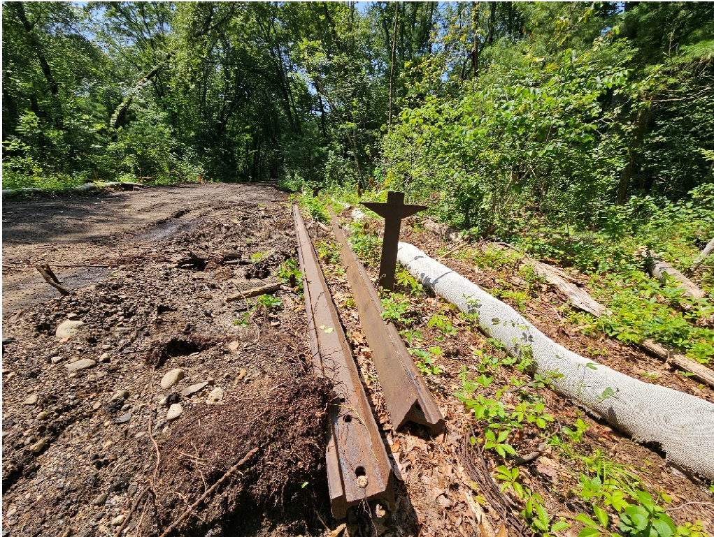
Photo 7. Existing rail and rail rests
