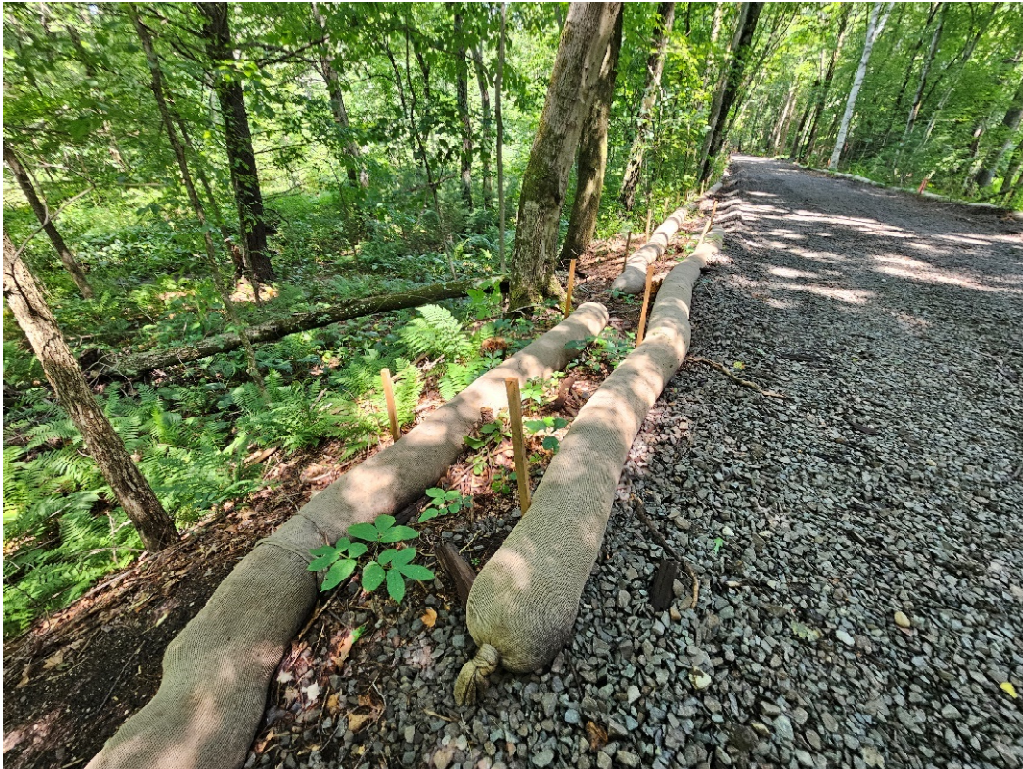
Photo 9. Sta. 227+25 RT: Syncopate sediment control barrier
