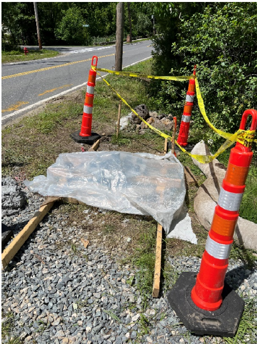
Photo 11: Sta. 307+80 looking at new HAWK signal foundation, standing at North Road
