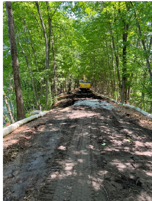
Photo 12: Sta. 321+50 looking north
