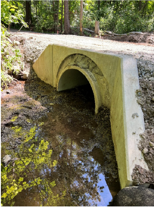
Photo 5: Sta 167+20 looking at new 48 inch culvert
