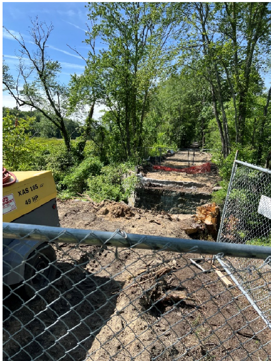
Photo 3: Sta. 126+50 looking south at Hop Brook
