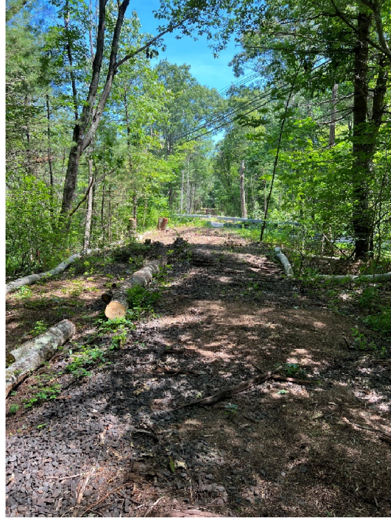
Photo 10: Sta. 283+50 looking north towards Pantry Road
