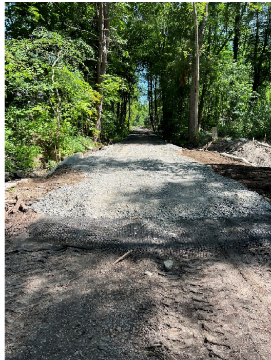
Photo 4: Sta. 167+00 looking north towards Hudson Road
