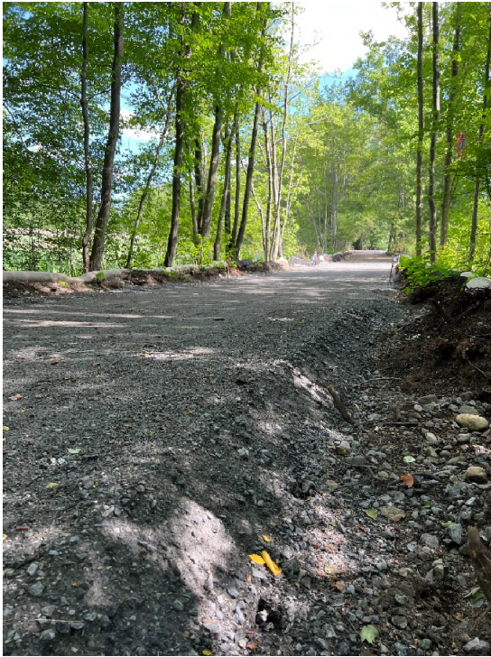
Photo 1: Sta. 104+00 looking north
