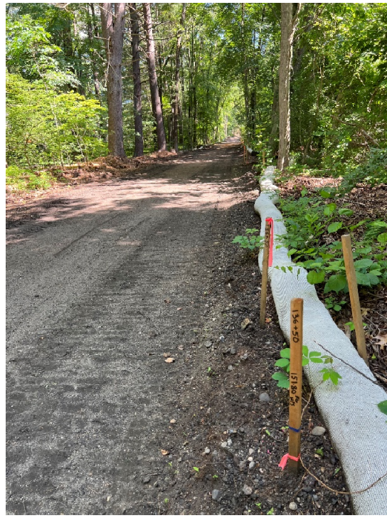
Photo 2: Sta. 136+50 looking north
