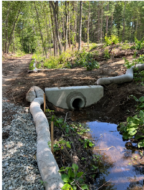
Photo 8: Sta. 216+50 looking north at new culvert
