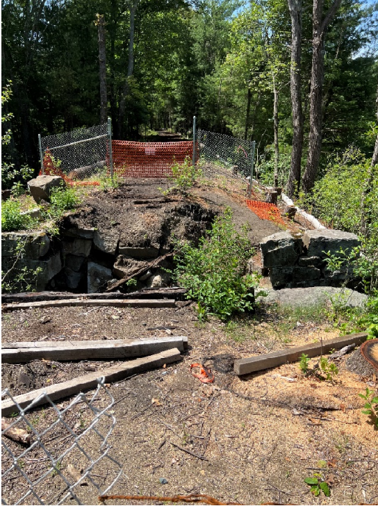
Photo 9: Sta. 265+00 looking south at Pantry Brook
