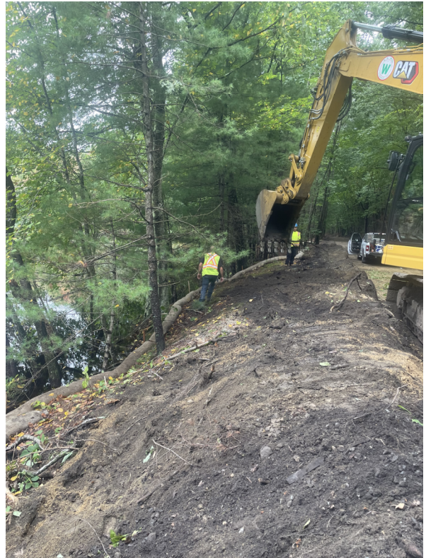
Photo 10. STA 332+00 looking North in between the wetland pond area and western limit of proposed trail. Side slope leading to pond appears to be in stable condition even after major rain events.
