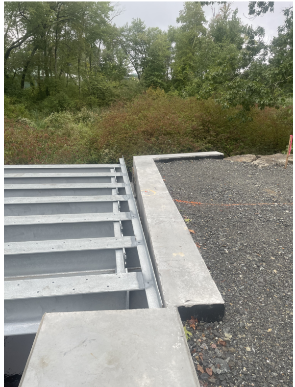
Photo 4: STA 191+00 facing East. Steel Structure erected at Hop Brook.
