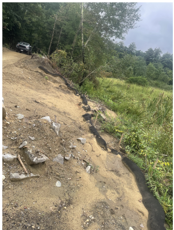
Photo 8: STA. 265+00 looking south at the side slope of Pantry Brook.
