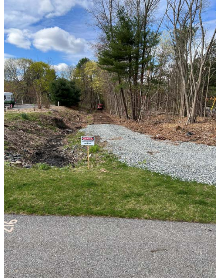
Looking South standing at Hudson Road
