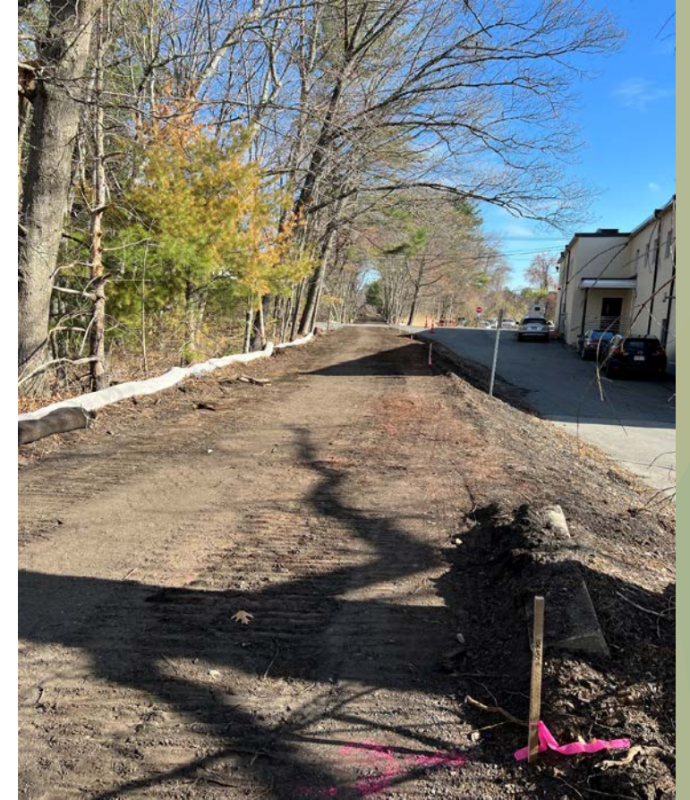
Looking North towards 71 Union Ave Driveway
