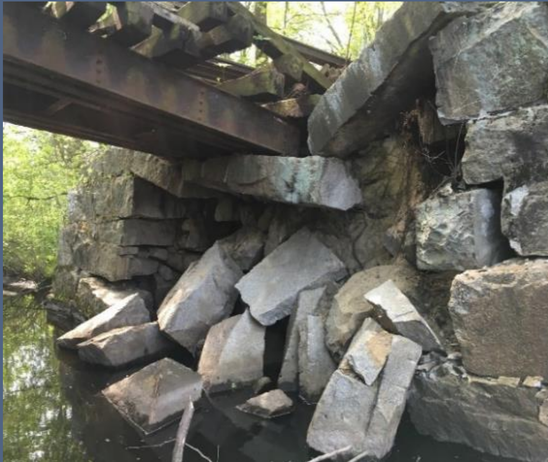
EXISTING PANTRY SOUTH ABUTMENT
