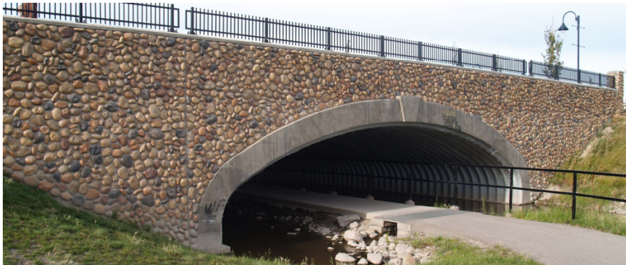
Example 1: Galv steel buried arch with aesthetic façade
