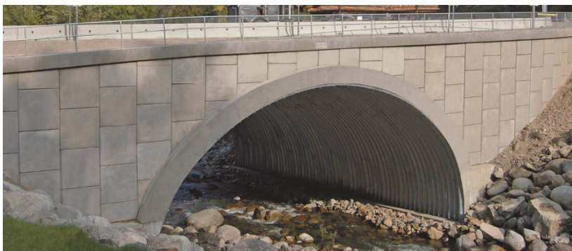
Example 2: Galv steel buried arch with aesthetic façade
