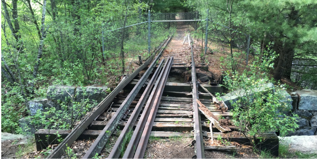
Looking South Across Bridge
