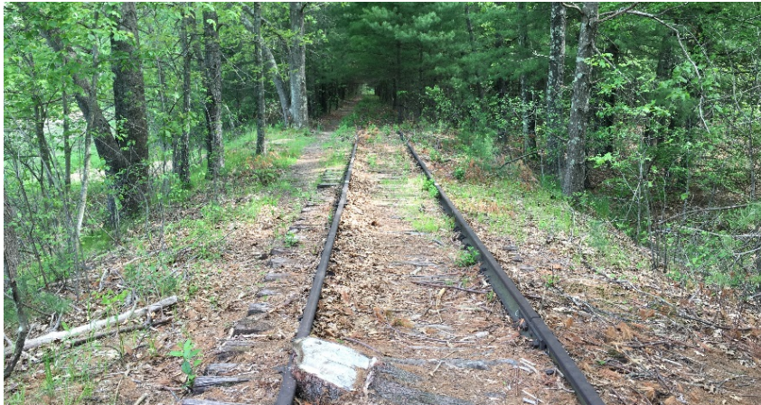
North Approach (Looking North)
