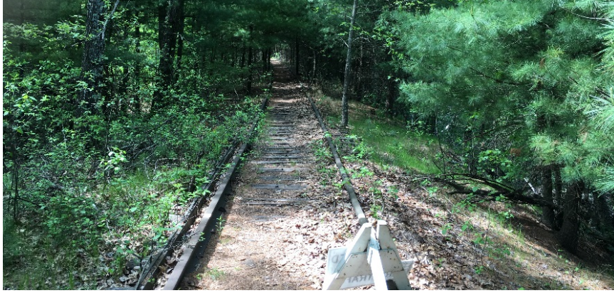
South Approach (Looking South)
