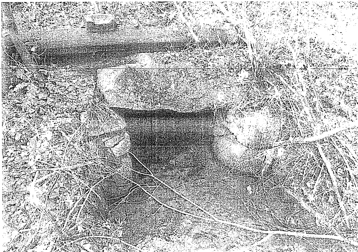
Photo 2 – Culvert under the old Railroad Bed (Analysis Point 6)
