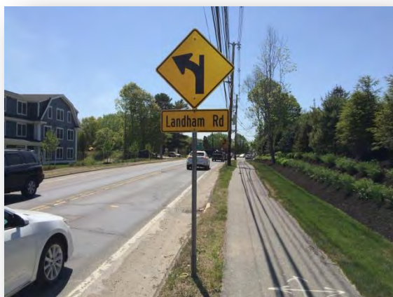
Existing W1-10b sign along westbound approach that does not properly portray horizontal alignment of roadway.
