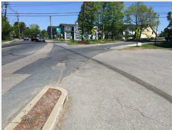
The wide and vague eastern driveway of Sudbury Auto. Inc. is located close to intersection adding additional conflict points.
