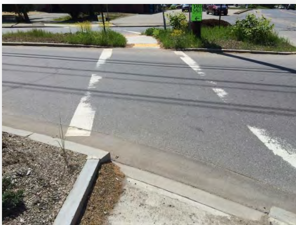
Crosswalks are significantly faded and debris is present within pedestrian refuge islands.
