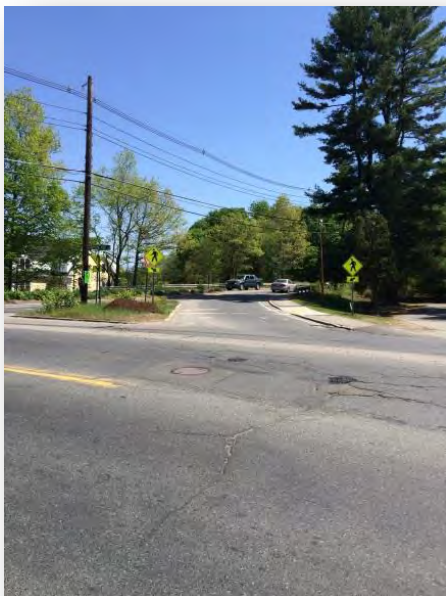
There is only one yield sign present for eastbound right turning land which is typically a fast turning movement.
