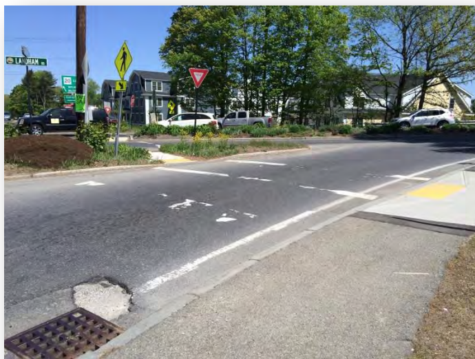
Slip lanes generally promote high speed turns which pose significant conflicts for pedestrians waiting to cross at these locations.
