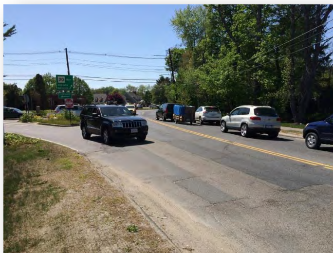
Westbound vehicles trying to pass left turning vehicles on the right which is very narrow and may result in a sideswipe collision.
