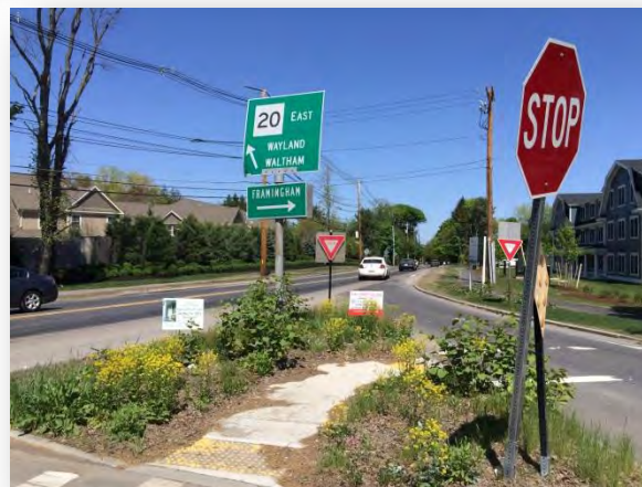
Green destination sign currently located in the eastern most island falsely directs motorists to enter Landham Road at wrong opening.
