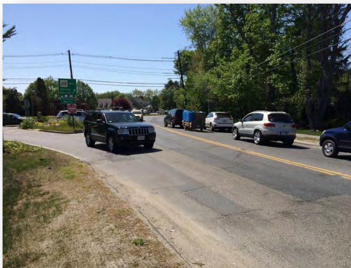
Queues develop along westbound approach on Route 20 as a result of left turning vehicle waiting for adequate gap in opposing traffic.
