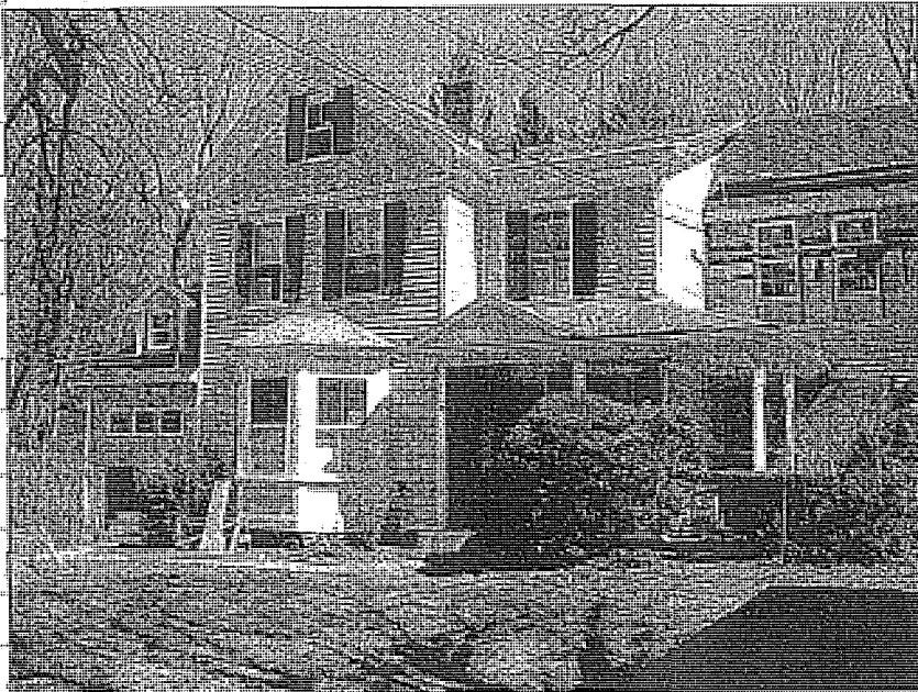
10 Maple Avenue – Spring 2006 – during construction
