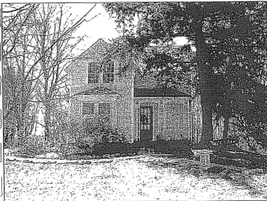
Main façade from road
