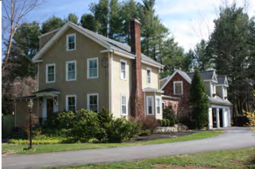
Façade (north) and west elevations.
