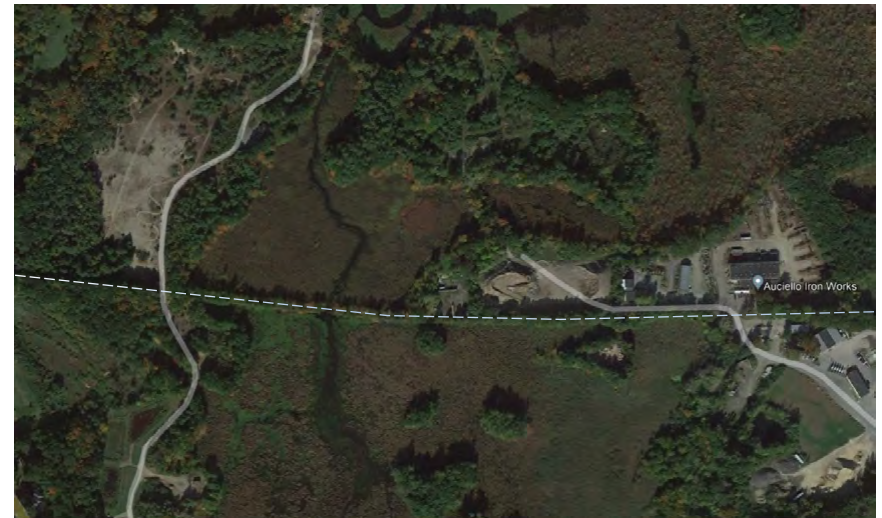
Fort Meadow Brook Crossing - Bridge #130 (Hudson - STA 149)
