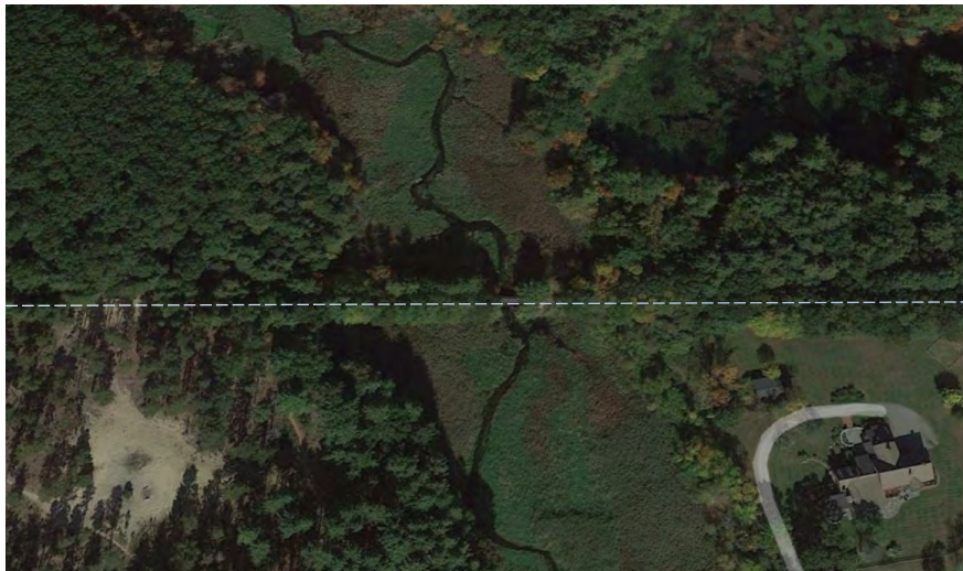
Hop Brook Crossing II - Bridge #128 (Sudbury – STA 400)
