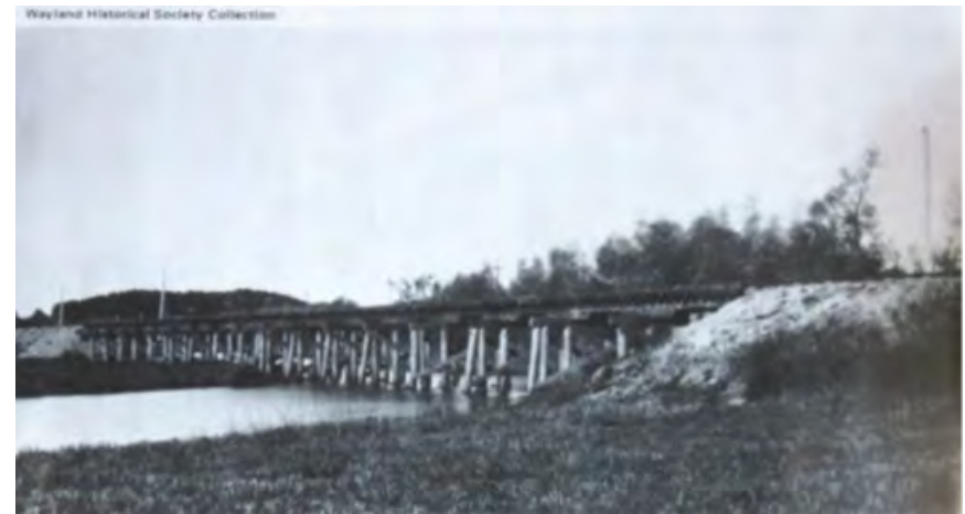
Trestle over Sudbury River west of Wayland in 1882. Note fill placed on original ground surface for the rail bed near waterways (Boston & Maine Hist. Society, 2008).
