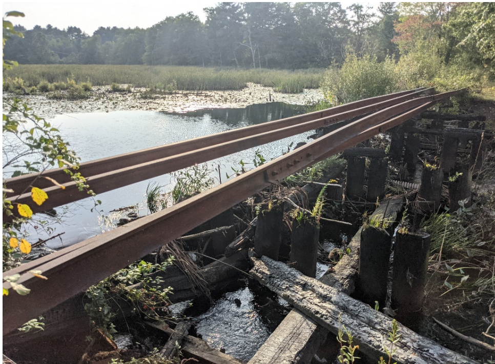
Photo # 11 Bridge 130 at MP 25.37, view southeast
