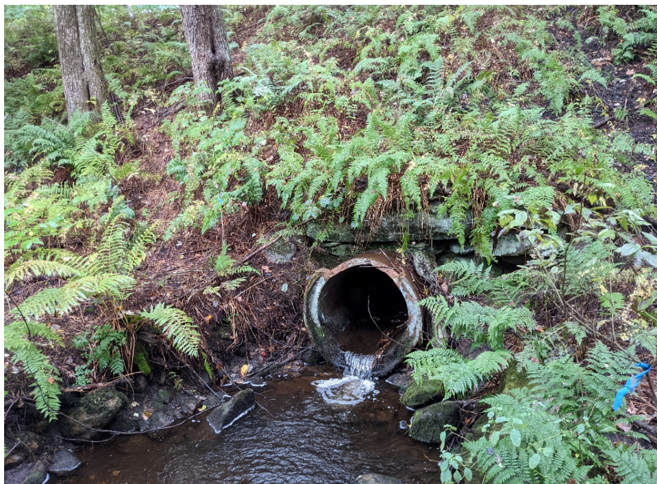
Photo # 13 Culvert 132A at MP 26.12, south end and embankment, view south
