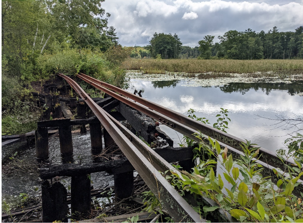
Photo # 10 Bridge 130 at MP 25.37, view northwest
