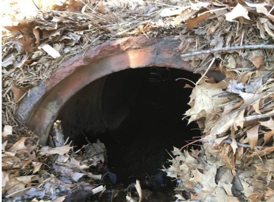
Photo # 12 Culvert 129C at MP 24.30, south end inlet, view north
