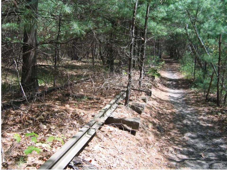
Photo # 2 Raised rail bed east of White Pond Road, view east
