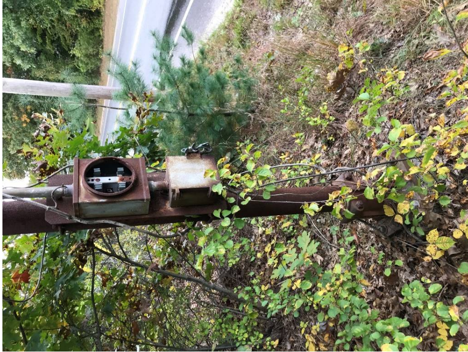
Photo # 20 Utility Pole at MP 24.76, view south
