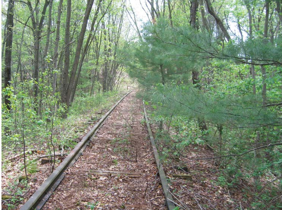
Photo # 8 Raised rail bed approaching Chestnut Street, view east
