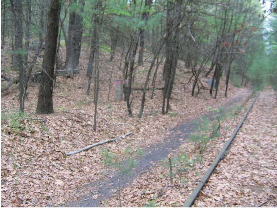
Photo # 4 Rail bed and knoll east of Parmenter Road, mile marker 23 visible on left (pink tag), view northeast
