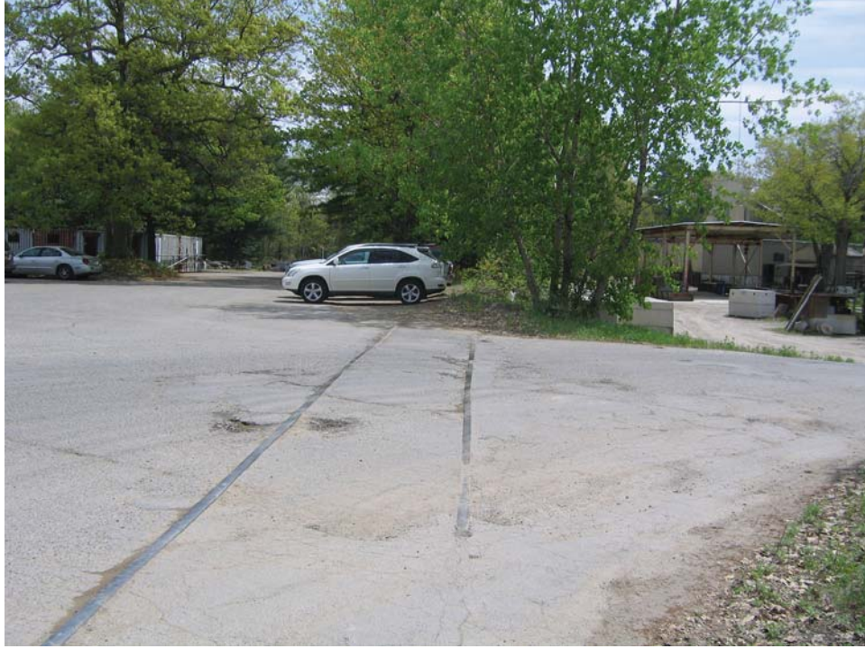
Photo # 6 Crossing at paved access road west of Main Street showing extant rails, view southeast
