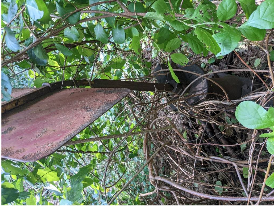
Photo # 42 Switch Stand and Electrical Box at MP 24.80, view south
