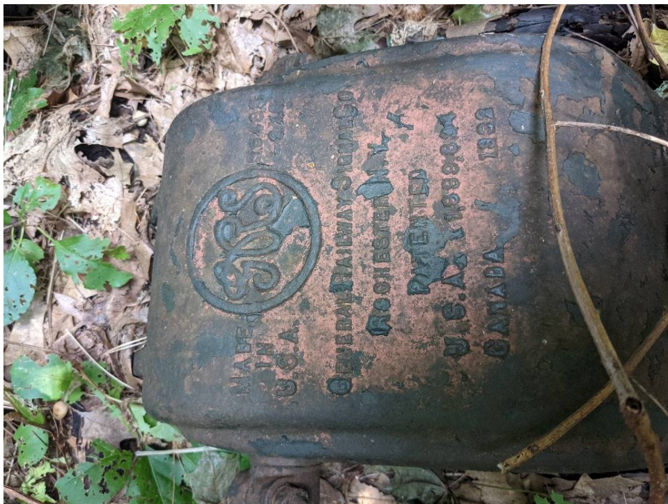
Photo # 43 Closeup of Electrical Box cover at MP 24.80
