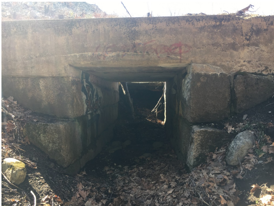
Photo # 17 Cattle Pass at MP 25.83, north side, view south
