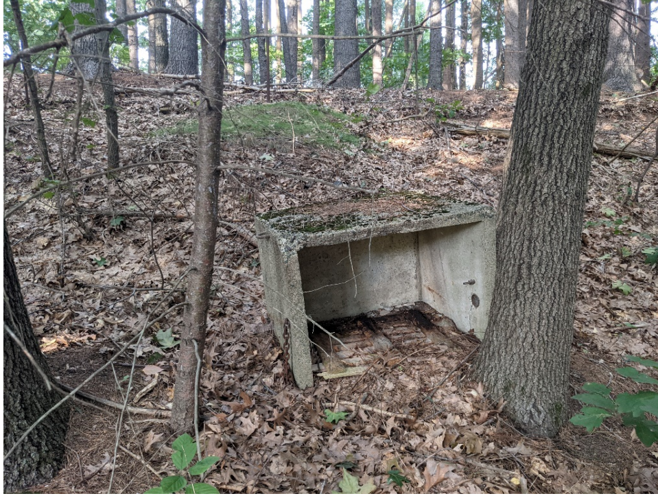
Photo # 22 Concrete mechanical/electric box at MP 24.89, view north
