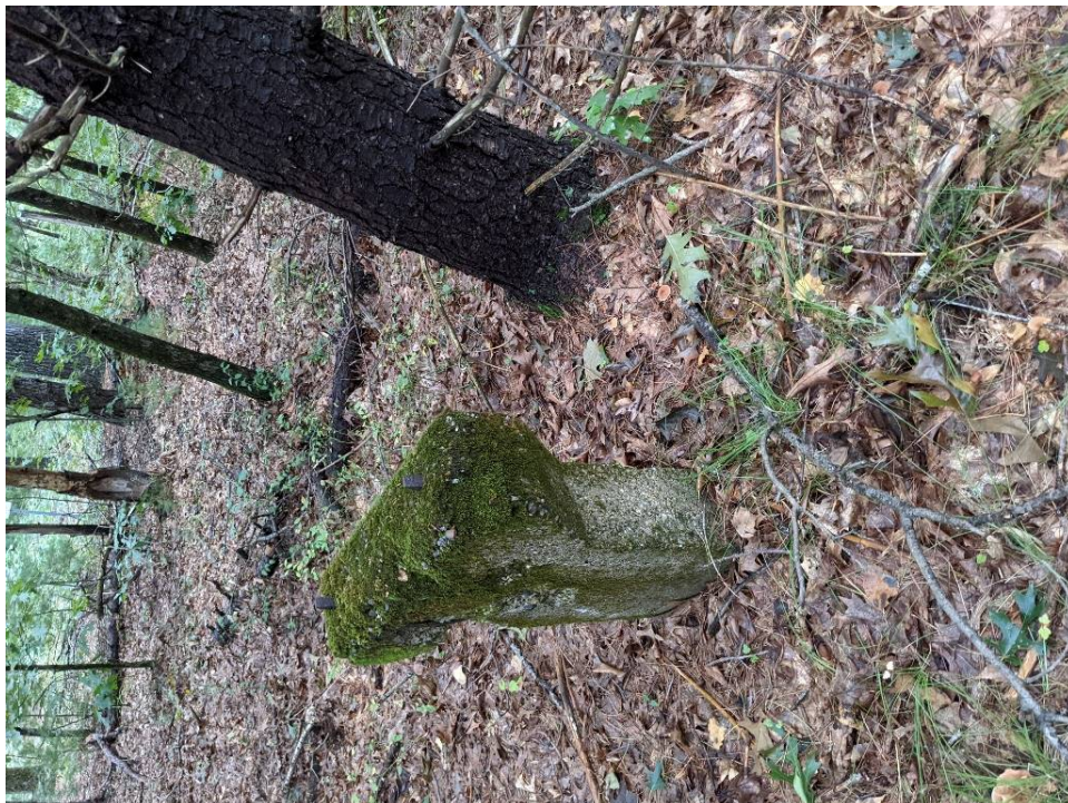
Photo # 35 Rail rest at MP 23.05, view southwest
