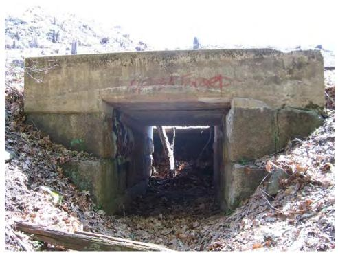
Plate 80. Partially buried concrete and granite block cattle crossing from orchard hill, view south.
