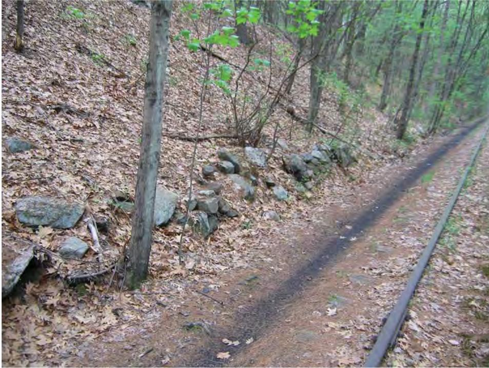
Plate 59. Railroad cut with field stone retaining wall, view east.
