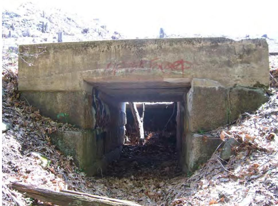
Plate 80. Partially buried concrete and granite block cattle crossing from orchard hill, view south.
