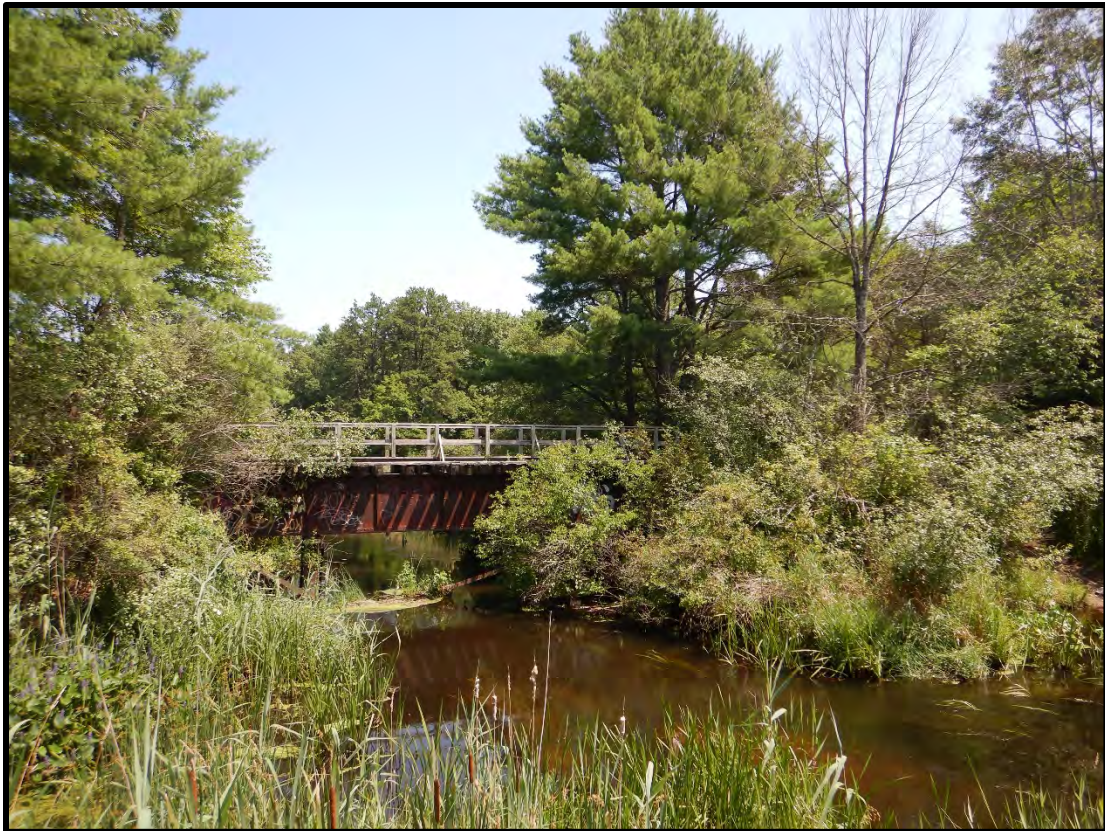
Photo 20 View of Bridge 127 over Hop Brook.
