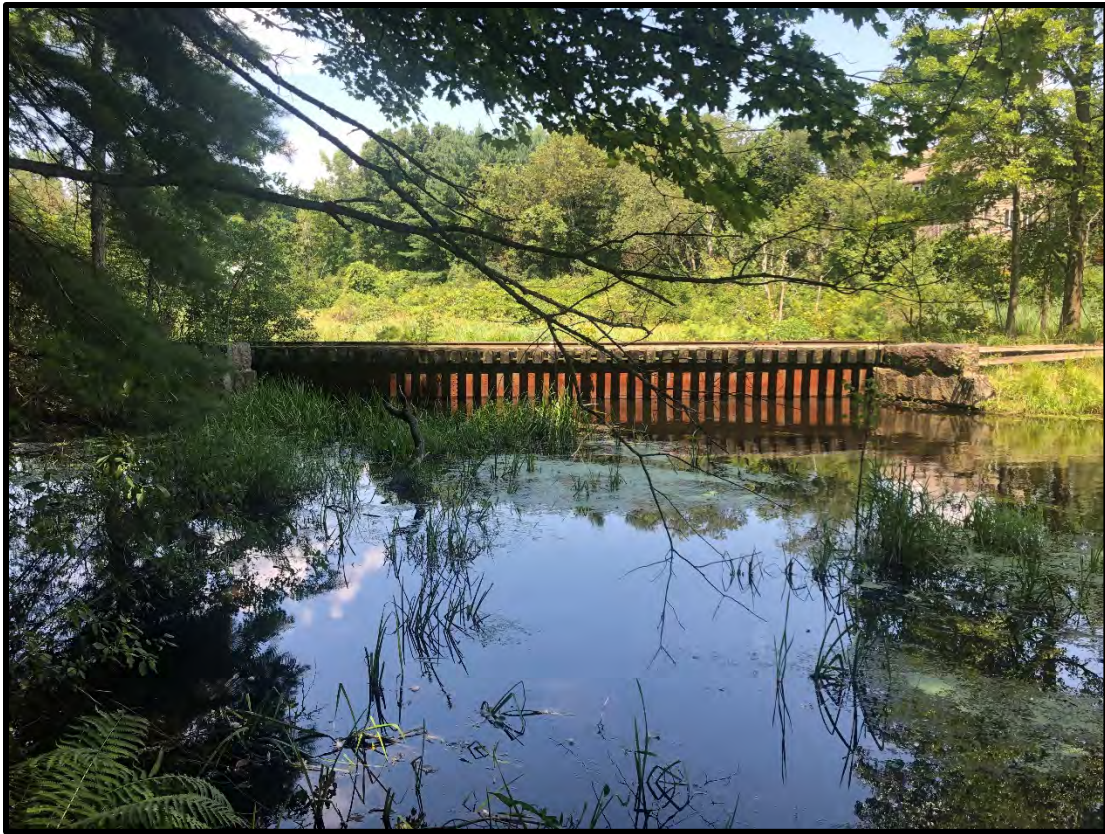
Photo 14 View of Bridge 127 over Hop Brook.
