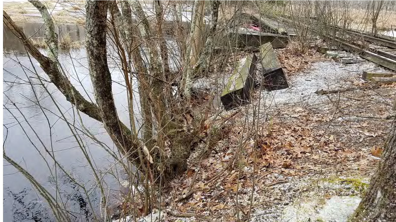
Photograph 9: Northwest side of Bridge 127. Heavily vegetated and steep slope.
