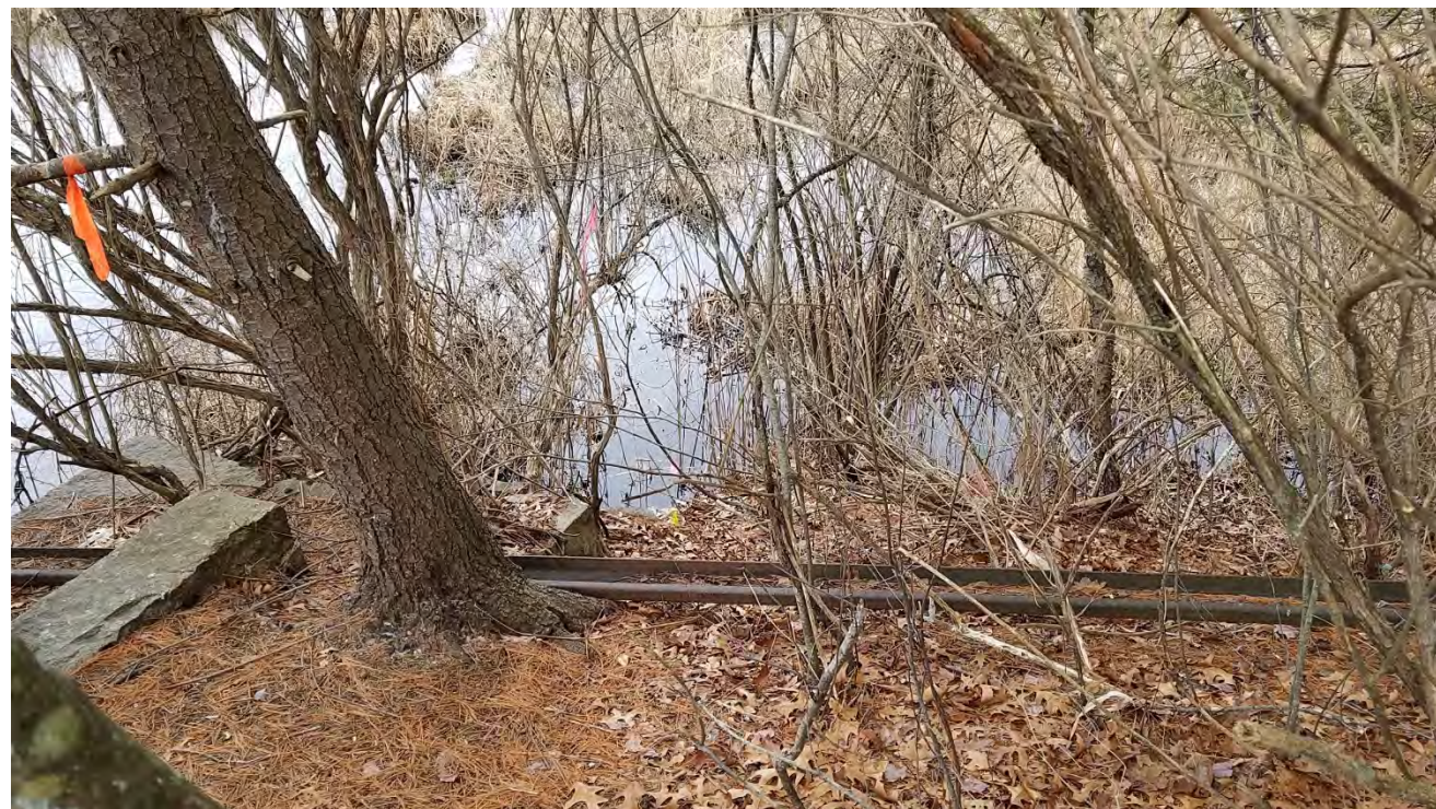
Photograph 7: Southwest side of Bridge 128. Heavily vegetated.
