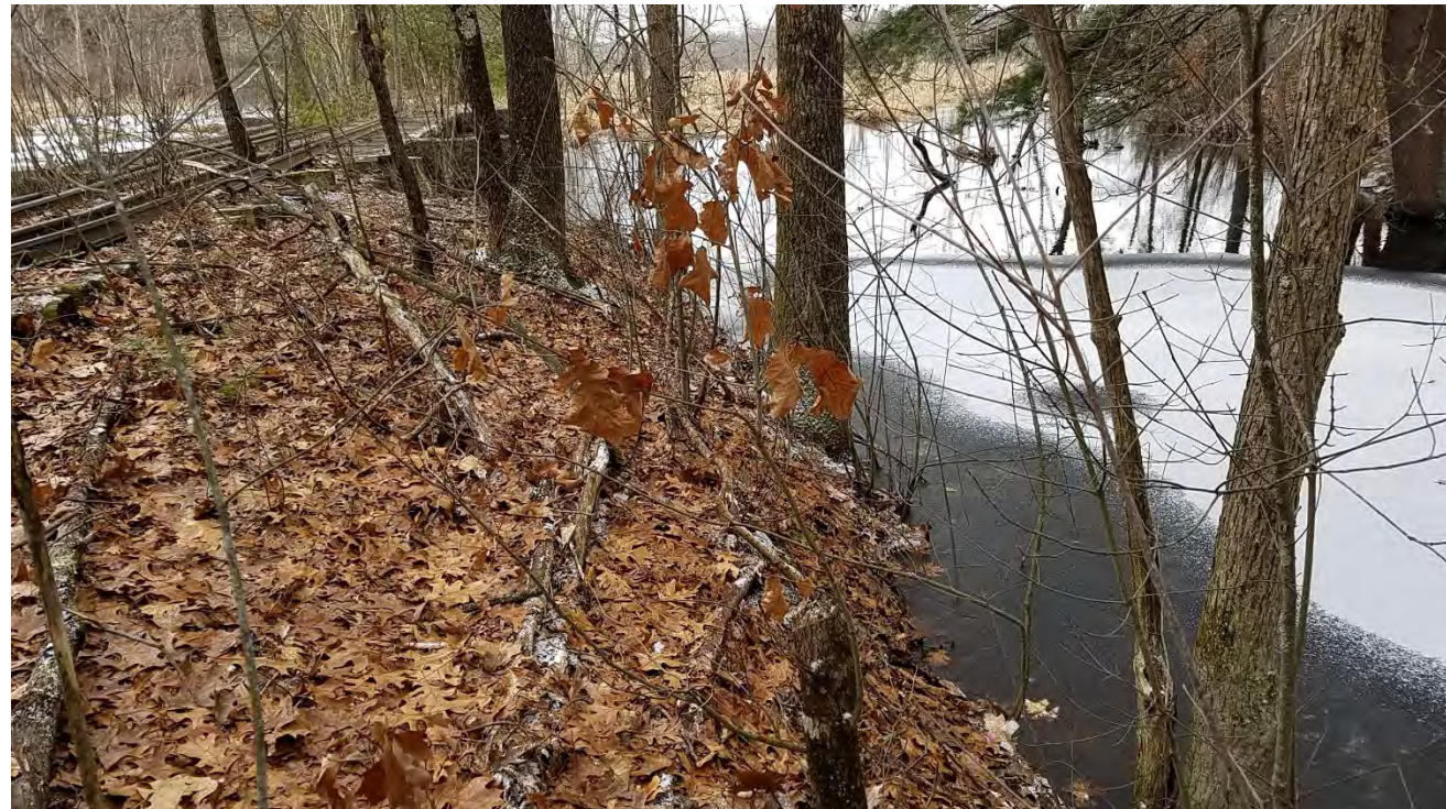
Photograph 11: Southwest side of Bridge 127. Steep slope.
