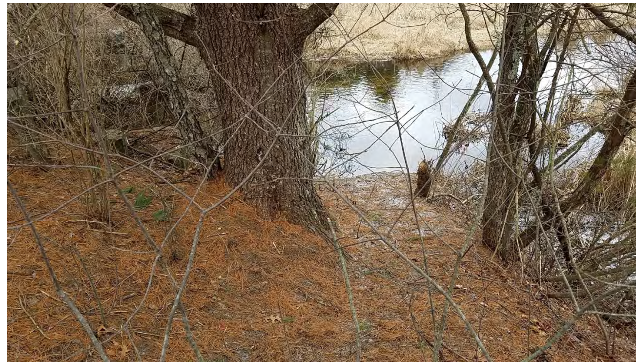
Photograph 6: Northeast side of Bridge 128. Portage here would result in minimal new impacts, as it is in the crane mat area, but impacts would be permanent rather than temporary.
