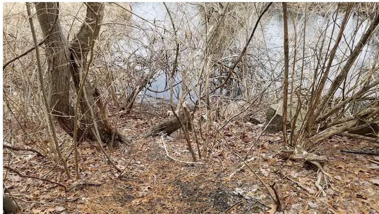
Photograph 5: Northwest side of Bridge 128. Heavily vegetated.
