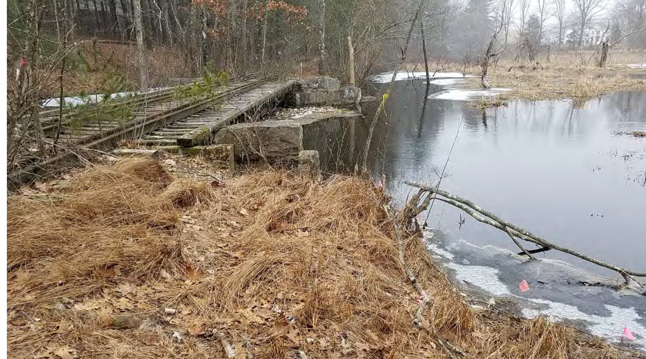
Photograph 10: Northeast side of Bridge 127. Gentle slope.
