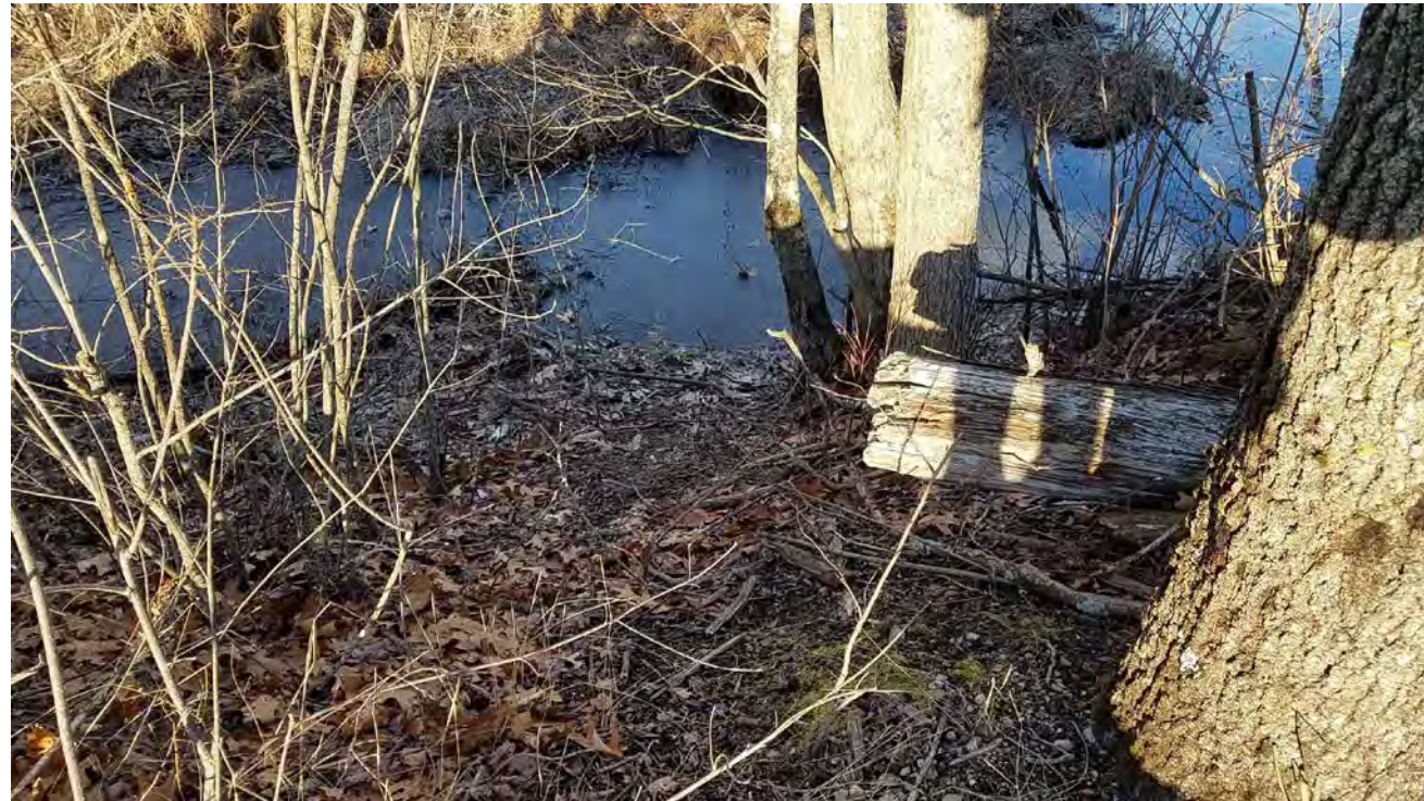
Photograph 1: Northwest side of Bridge 130. Heavily vegetated and steep slope.
