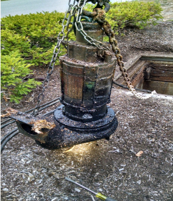
Existing Septic Pump
