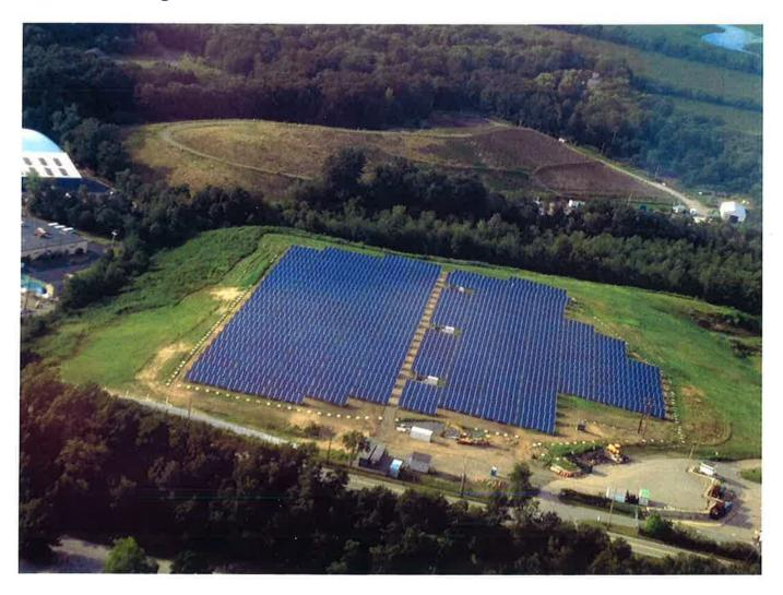
Sudbury Solar One facility located at Sudbury's closed landfill. Completed in November 2013, this 1.5 MW solar farm will generate 1.9 million kWh from more than 6,000, 250-watt modules on the site.
