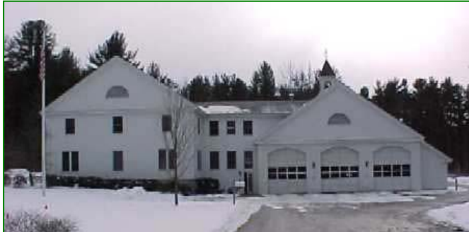
Sudbury Fire Headquarters
