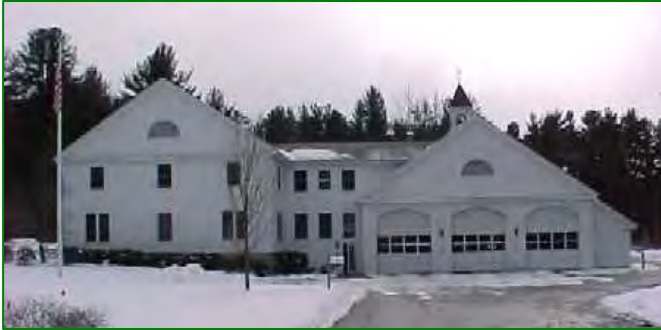
Sudbury Fire Headquarters
